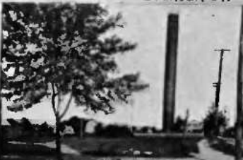
STAND PIPE WATER WORKS
