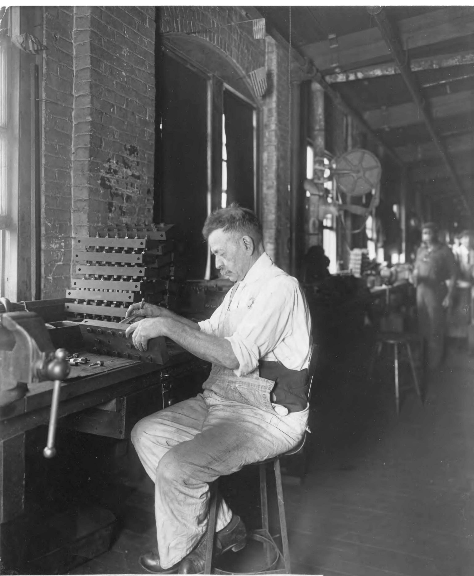
#15 Blind Man Assembling Starter Contact Boards. Crocker-Whooler Co., Ampero, N. J.
