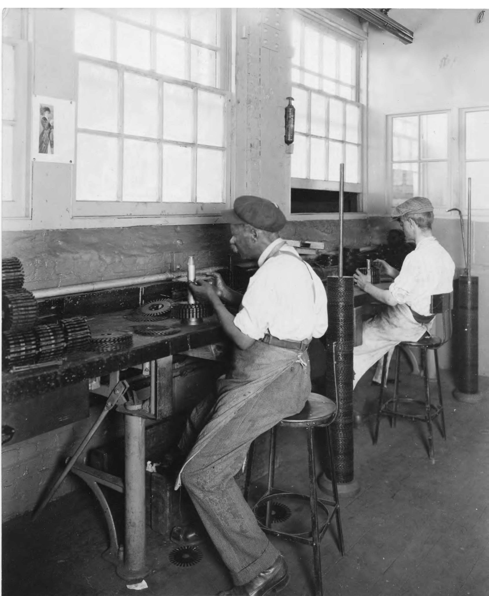
#11 Blind employees Assembling Armature Cores. Crocker-Wheeler Co., Amperc, N. J.
