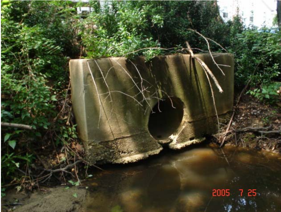
Figure 10: Outfall on the West Branch of the Pompeston Creek Draining Residential Area
