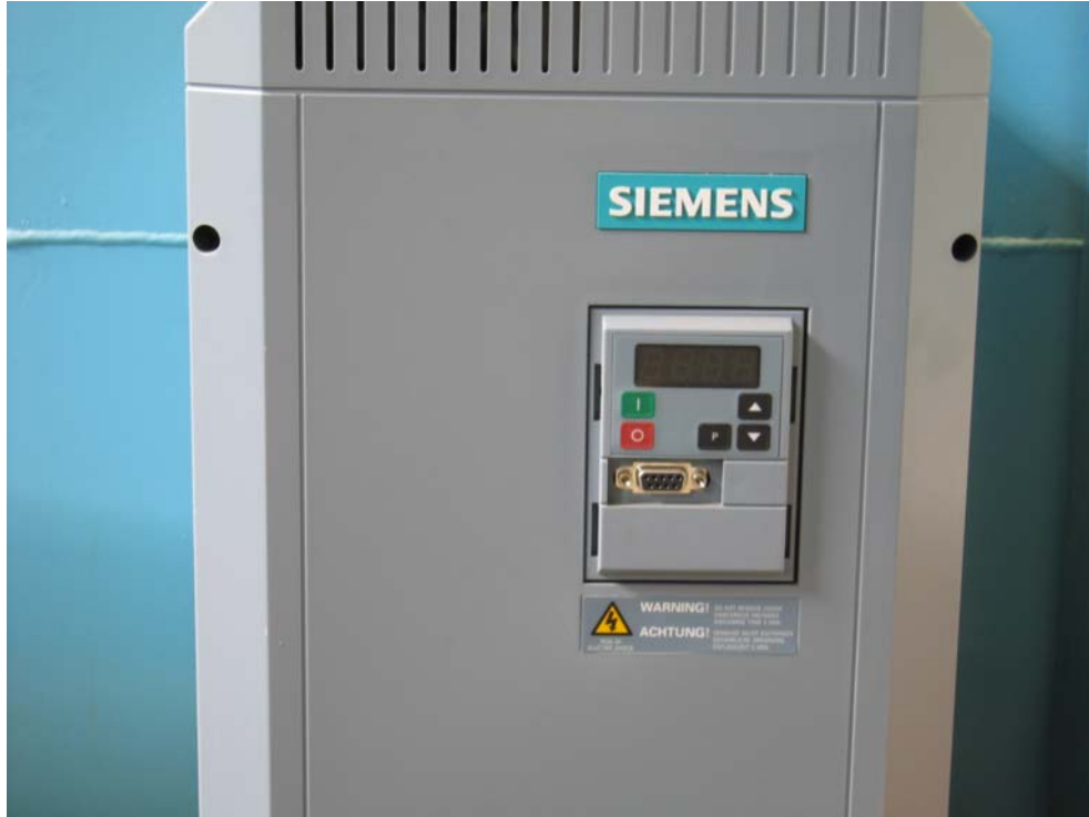
Figure 2.2: Siemens Midimaster Eco variable frequency drive
