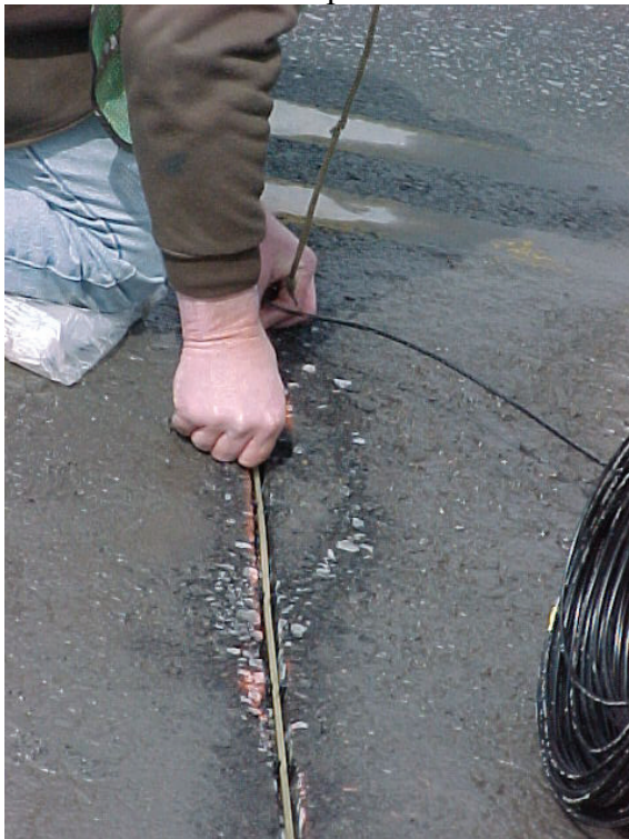
(c) Step 3 – Place piezo sensor into slot
