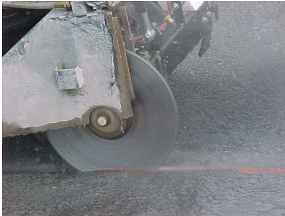
(a) Step 1-cutting slots for piezo sensors and loops
