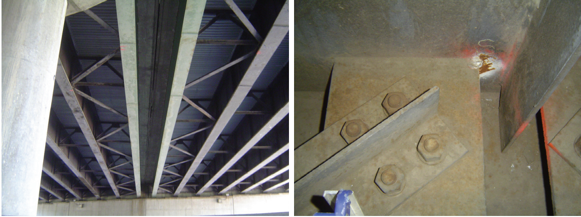
Figure 4.34 Route 202/23 bridge: (a) under deck view of girders and bracing and (b) close-up view of lateral connection plate and cracked web
