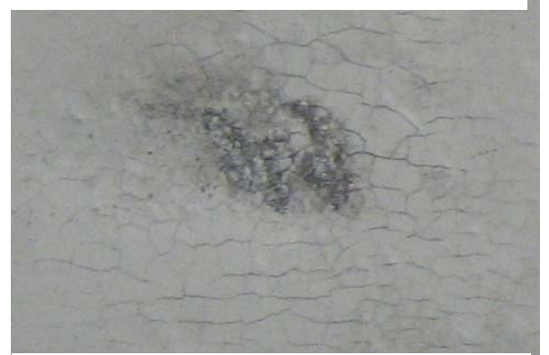
Fig. 3.3.2 shows large cracks under visual observation
