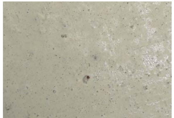
Fig. 3.10.2 shows depressions and holes in the surface
