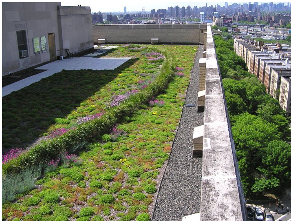
Figure 1. Green roof on the Bronx Courthouse. Photo May 16, 2007, Kate Shackford, BOEDC.
