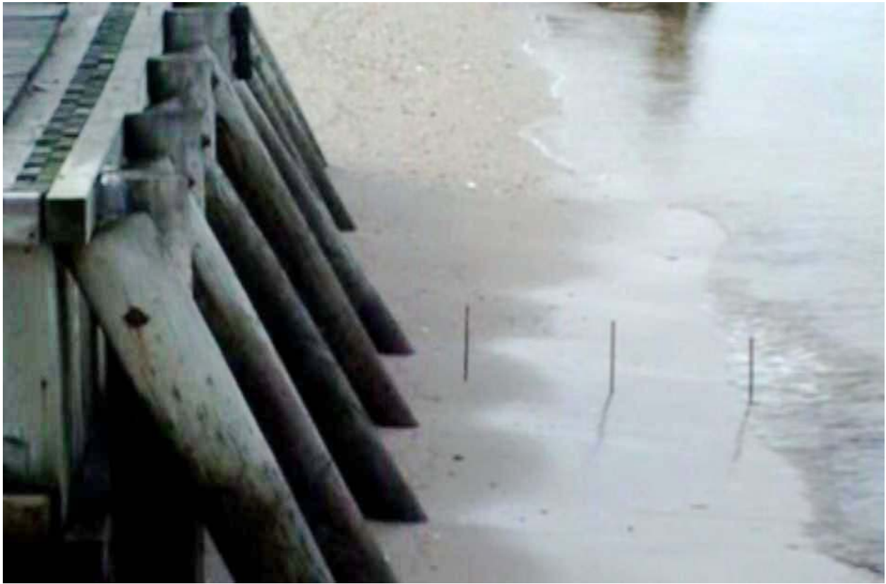
Figure 9 The differential drainage in front of the north bulkhead.
