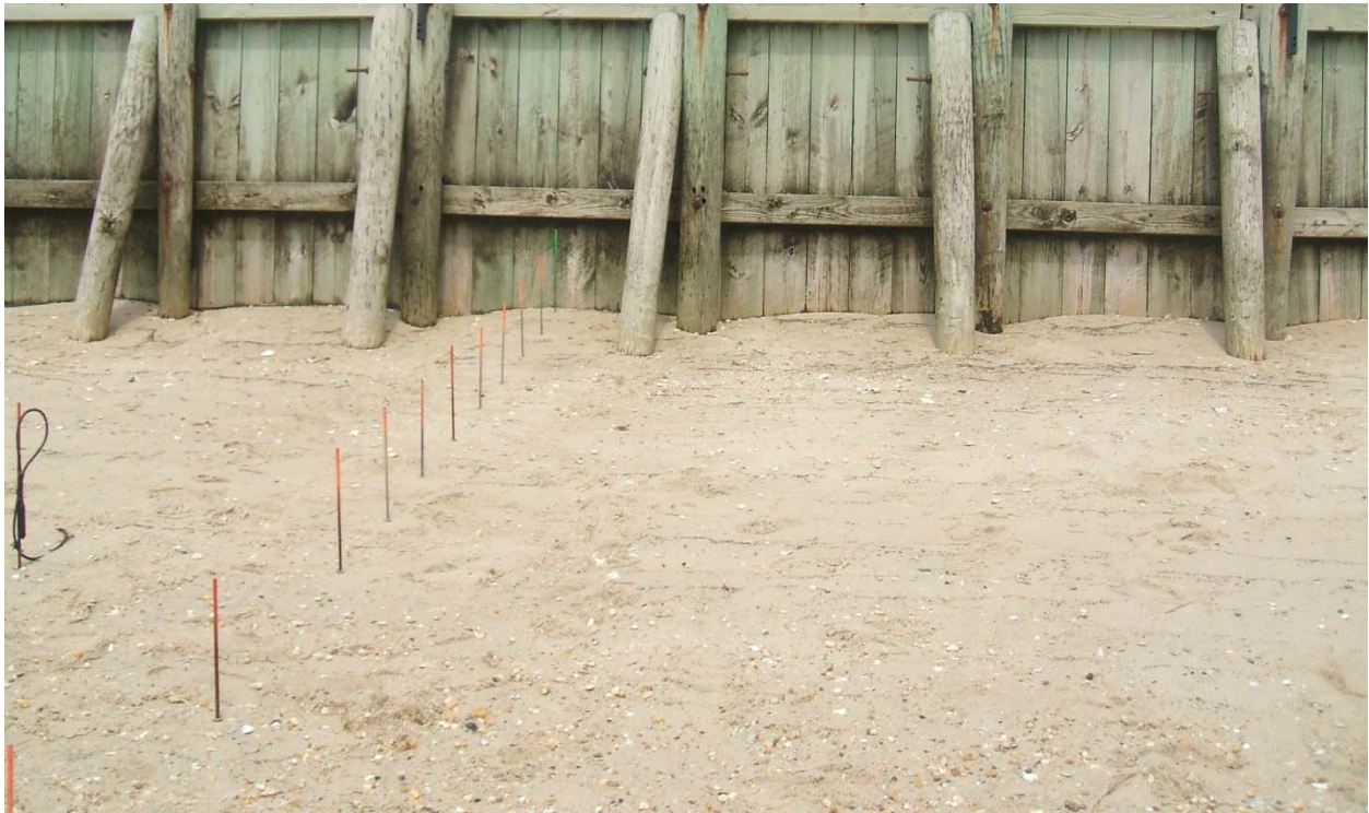
Figure 10 The alongshore topographic variability in front of the south bulkhead is irregular, with mounds in front of the planar sections of the bulkhead. Also evident is the decrease in surface elevation from south to north.
