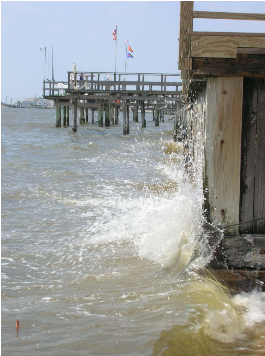
Figure 11 Jets of water produced during rising tide at the north bulkhead as waves break in front of or at the bulkhead and water is trapped between the wall and lower gunwale.
