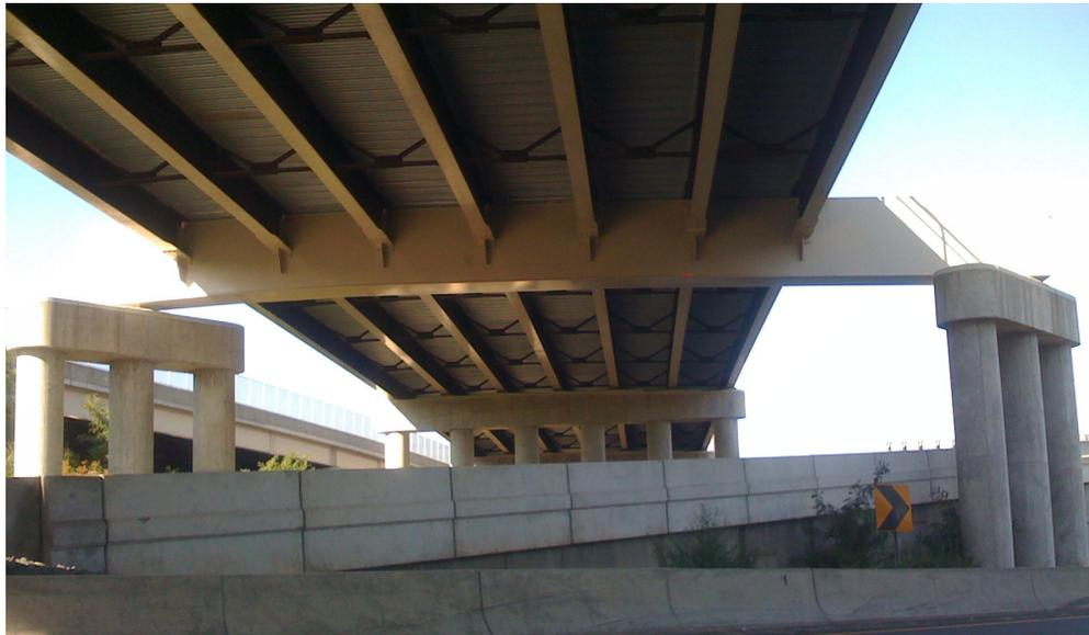
Fig. 6.6. Multiple column straddle bent (Route 130 East Brunswick, NJ)
