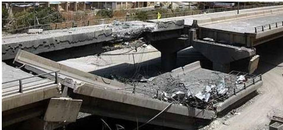
Fig. 2.10. Collapse of bridge due to blast (courtesy AFP / Getty Images)
