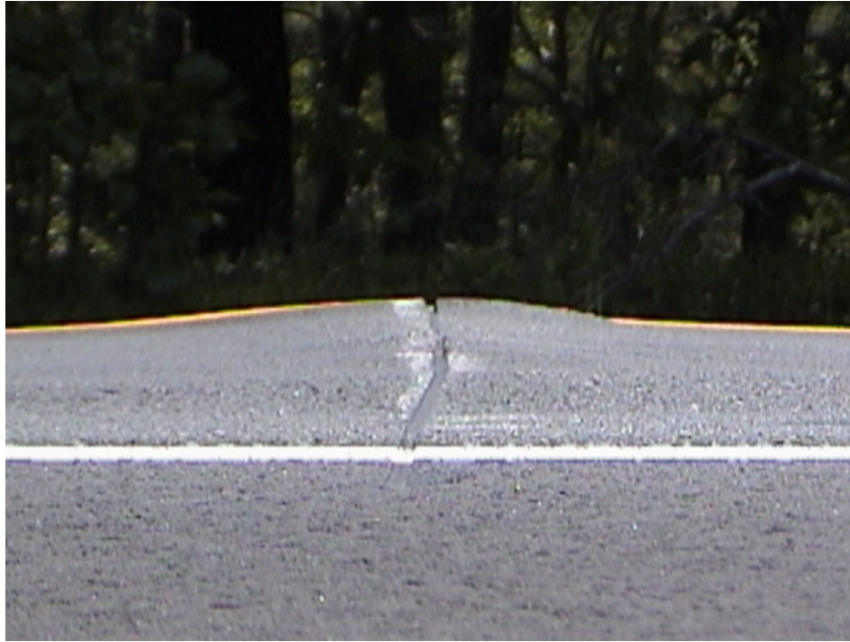
Figure 2.4 – HMA Overlay Failure at Joint Area Due to Excessive Curling Forces (Route 34 MP 11.5 Southbound)
