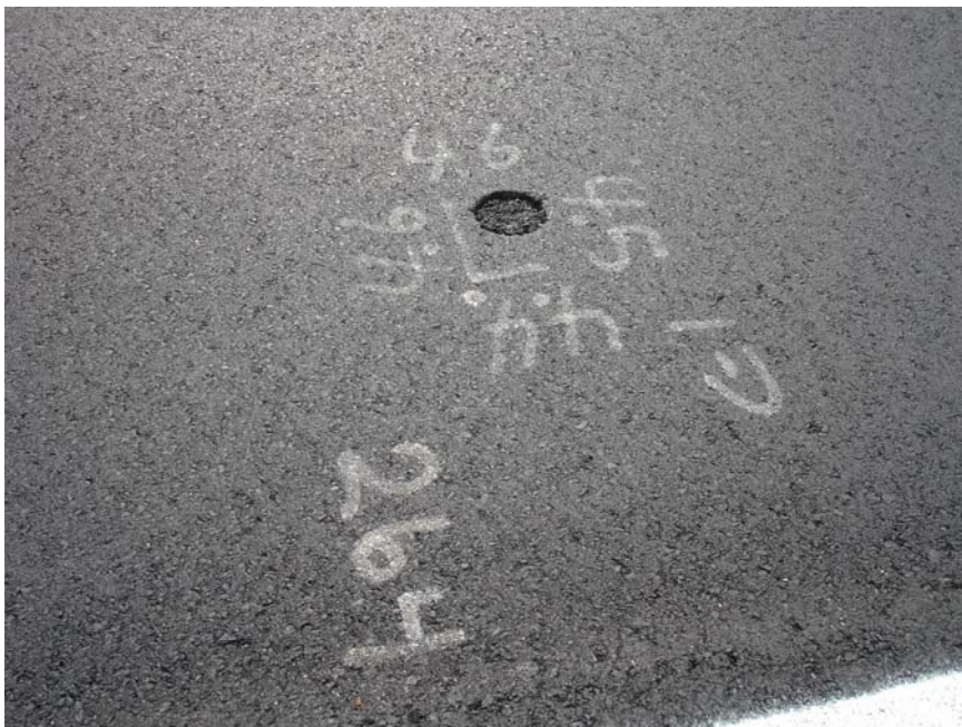
Figure 5.26 – Poor Backfilling of Extracted Core from Rt 202S in New Jersey
