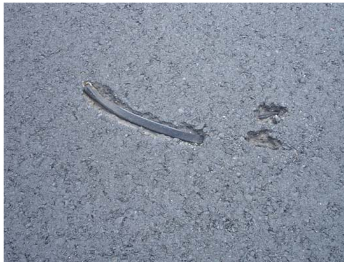
Figure 5.25 – Rubber Cord Paved into Pavement Surface of Rt 202S in New Jersey
