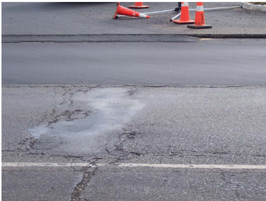
Figure 5.2 – Photo of Reflective Crack Relief Interlayer (RCRI) Mix, shown in far lane, and Existing HMA Patch Over Deteriorated Reflective Crack
