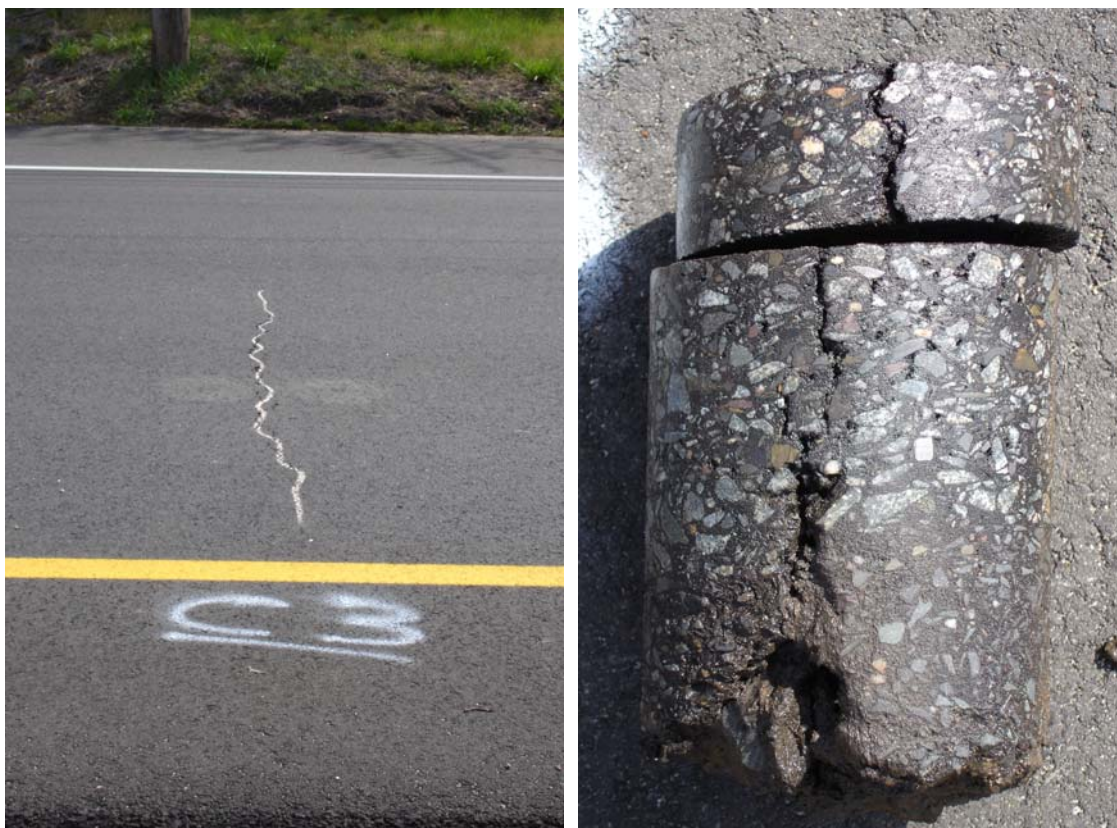
Figure 5.14 – Early Reflective Cracking in Test Section MP 2.5 to 4.5
