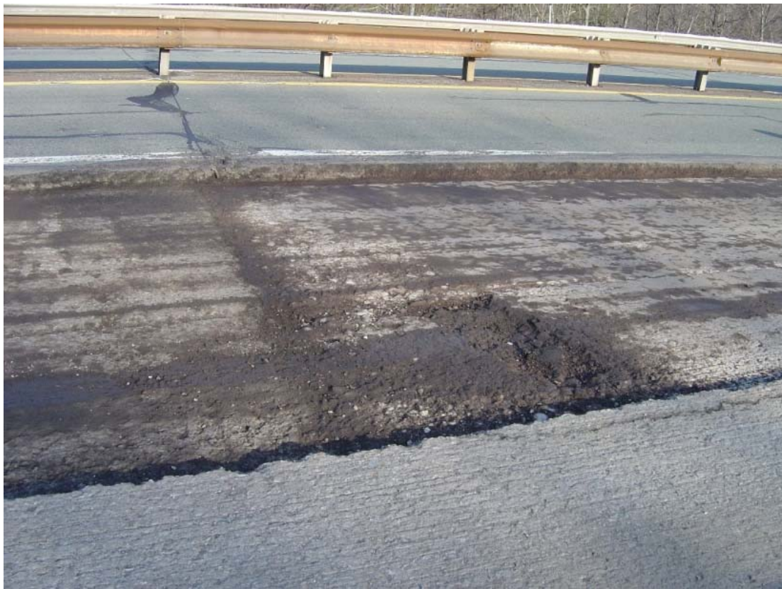
Figure 5.36 – Milled and Unmilled Surface of Interstate 476 in Pennsylvania
