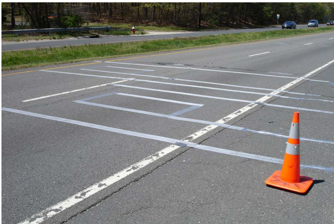
Figure 4.2 – Weigh-in-Motion/Automated Vehicle Classifiers (WIM/AVC)
