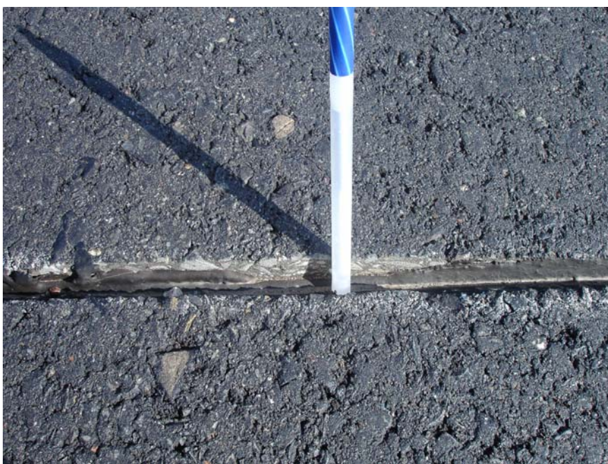
Figure 5.26 – Poor Backfilling of Extracted Core from Rt 202S in New Jersey
