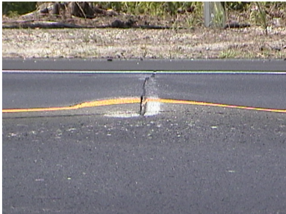
Figure 2.5 – HMA Overlay on Route 34 (Picture taken from Northbound Side showing the joint was only sawed and sealed on the Southbound Side)
