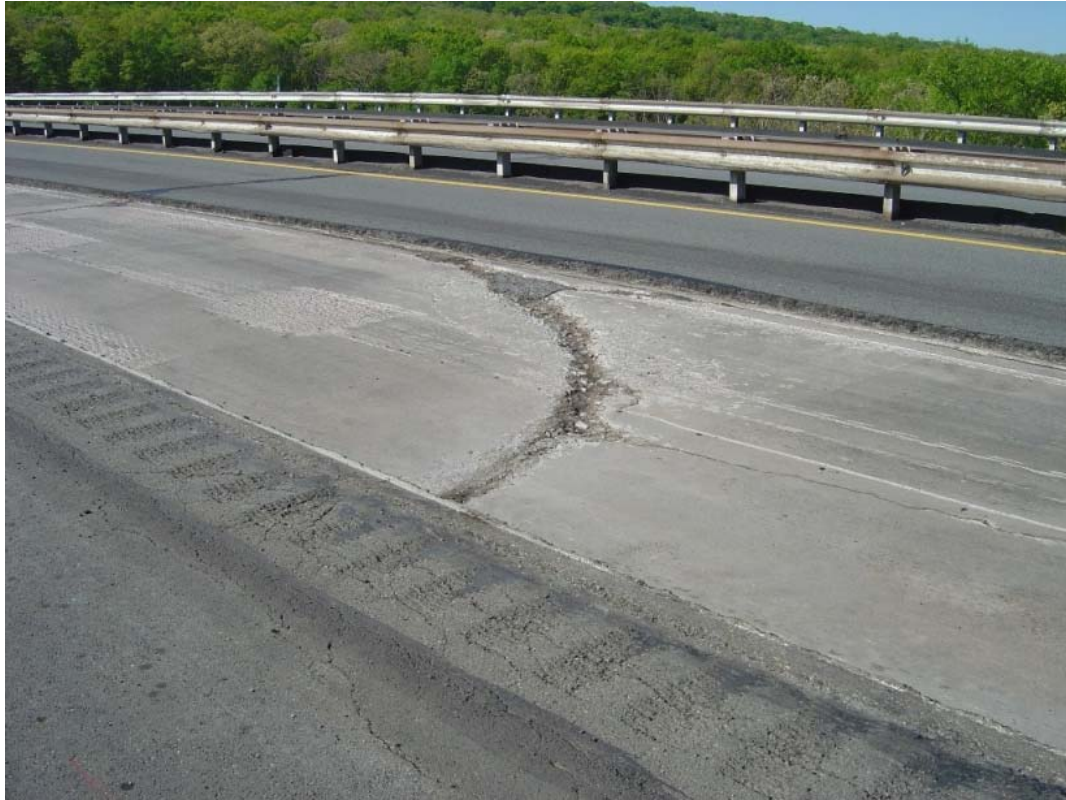
Figure 5.37 – Exposed Surface of Underlying PCC Pavement on Interstate 476 in Pennsylvania
