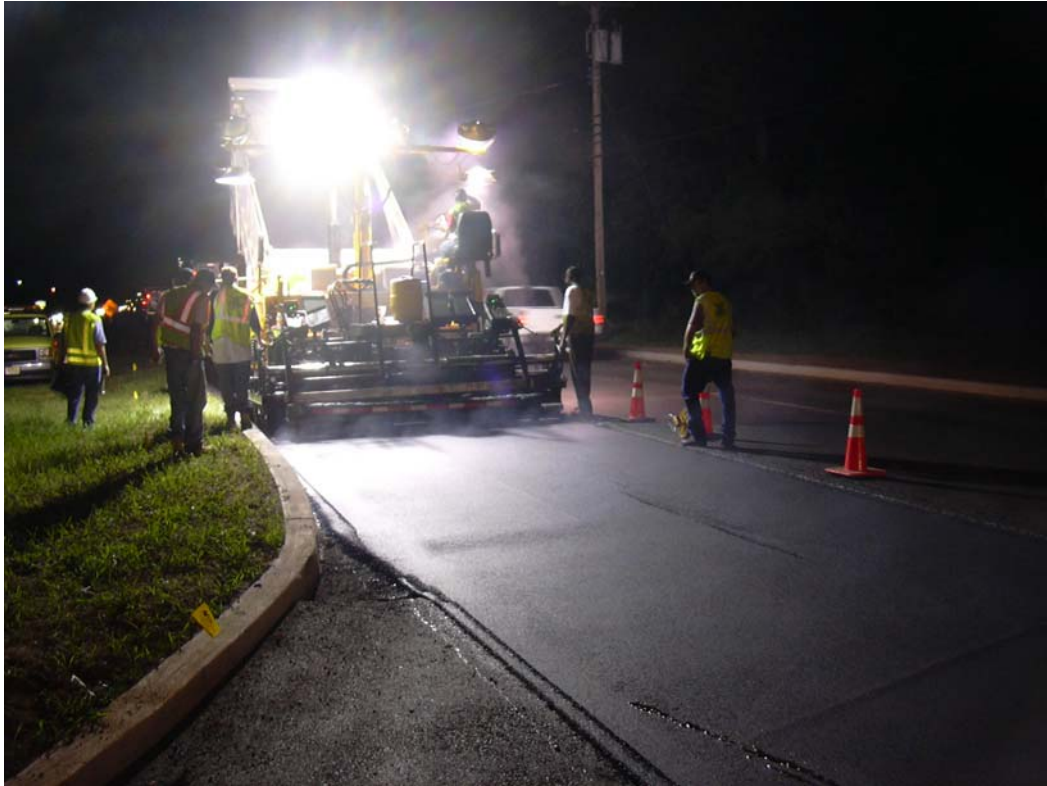
Figure 5.3 – Paving RCRI Mixture on Rt 34N in New Jersey
