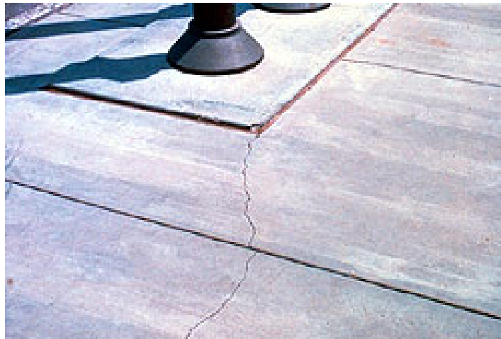
Figure 2-4: Drying shrinkage cracks
