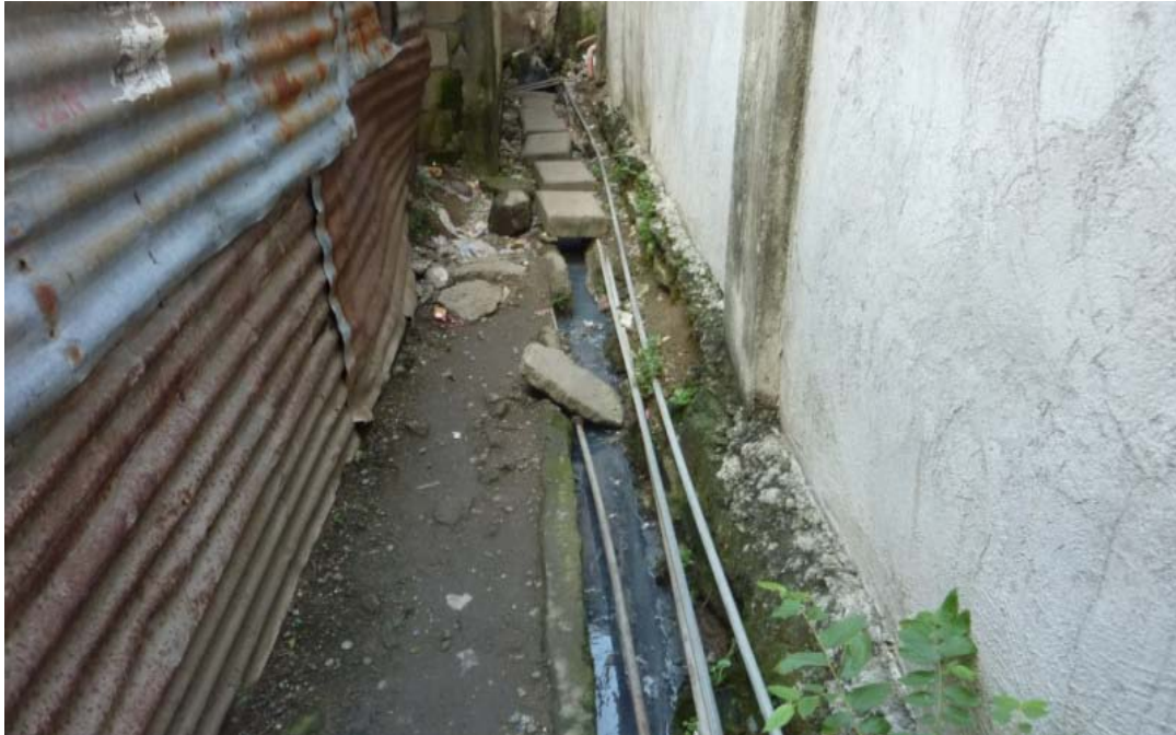
Figure 9.2 Damaged MCWD water distribution lines in open sewage canal in barangay Labangon
