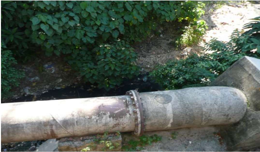
Figure 9.4 MCWD water-main in open sewage canal in barangay Labangon
