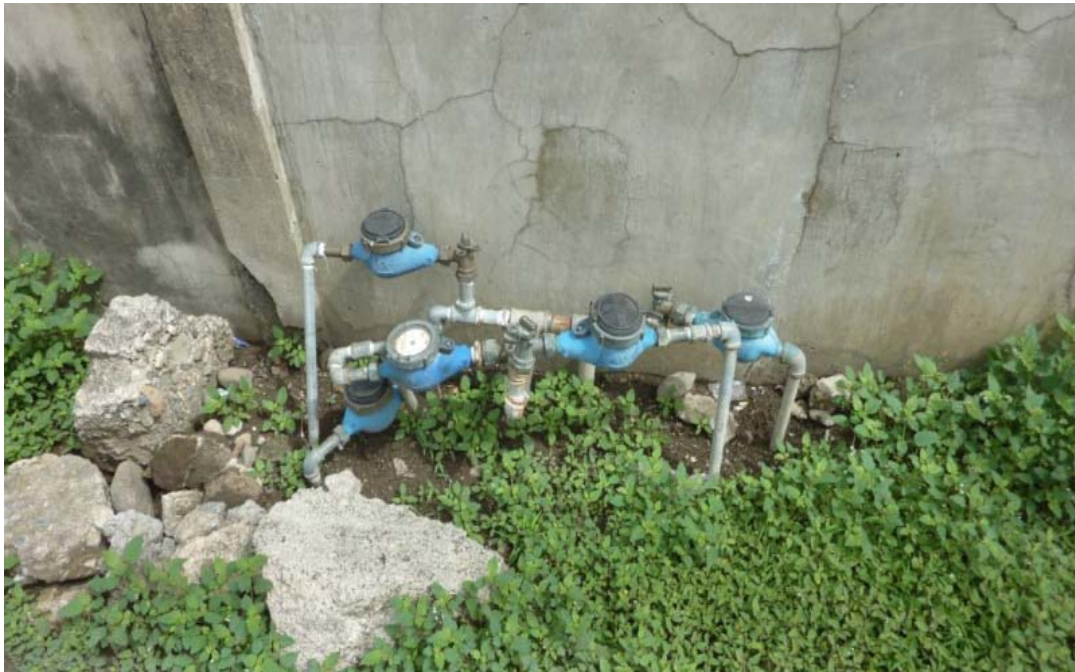
Figure 9.1 New water meters installed by the MCWD in barangay Labangon
