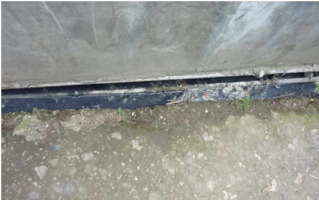
Figure 9.3 Partially submerged MCWD water distribution lines in open sewage canal
