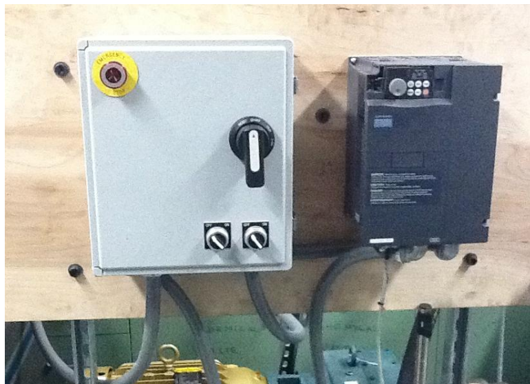
Figure 57: Electrical circuit breaker box (left) and Mitsubishi VFD (right). The circuit breaker box has emergency shut off (upper left), circuit throw level (middle right) and power switches for VFD (lower left) and power pack (lower right).
