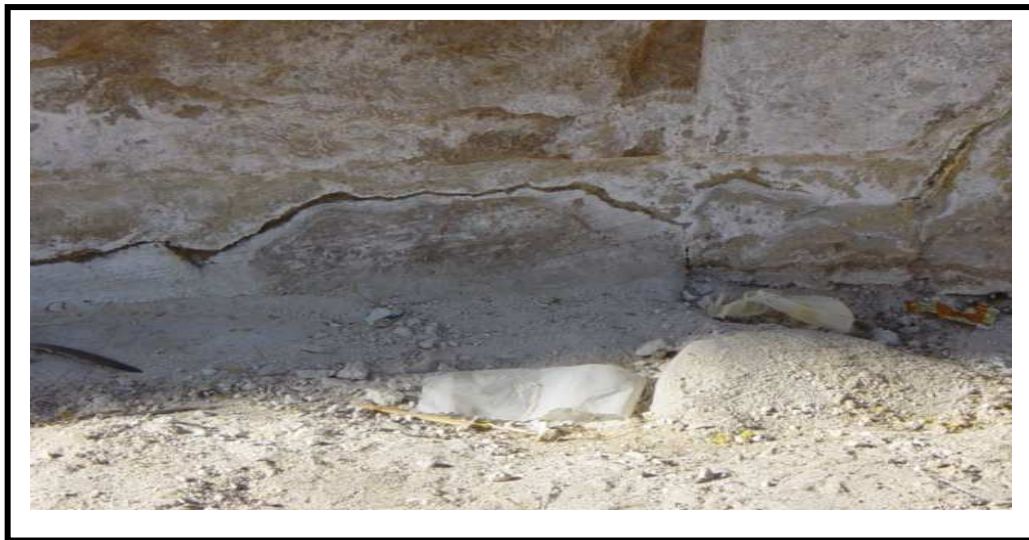
Figure 2: Effects of shallow saline groundwater on the Habu temple (note the severe cracks and salt accumulations)
