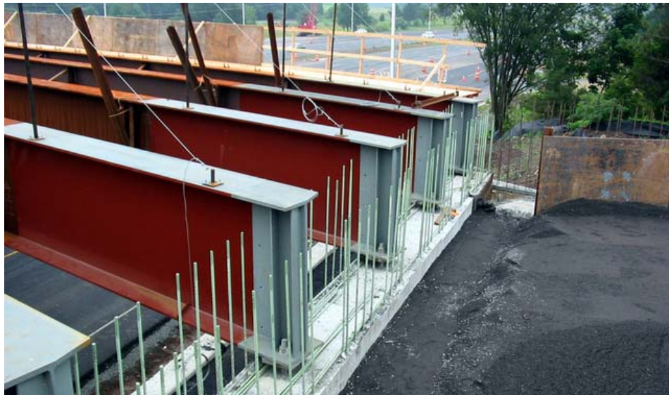
Figure 5.9 Abutment- Girder Connection (Courtesy of ARORA and ASSOCIATES, P.C)
