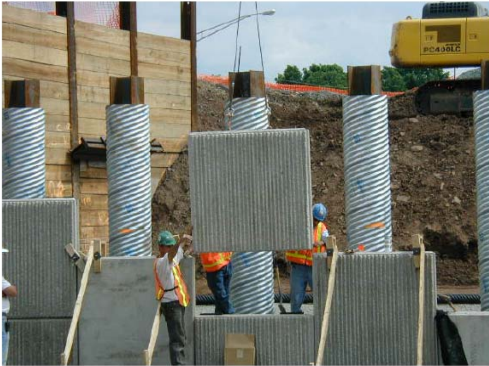
Figure 5.7 H-Piles Enclosed by Aluminum Sleeves (Courtesy of NJDOT)
