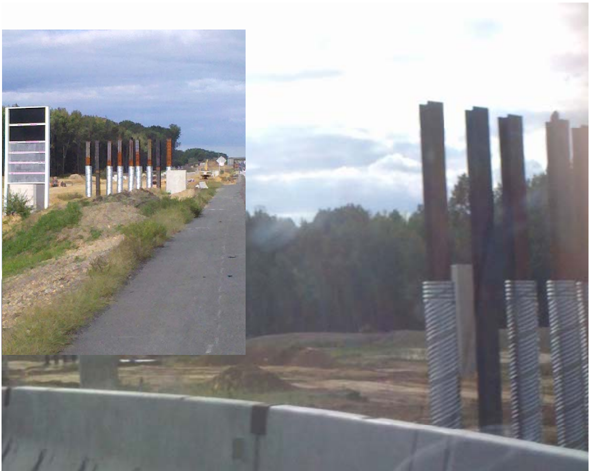
Figure 2.5 Sleeves Surrounding H-Piles at a Construction Site in New Jersey
