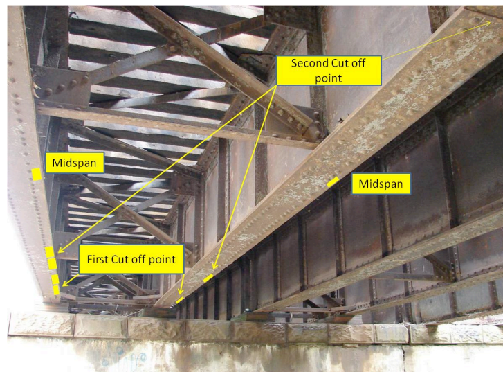
Figure 16. Bottom view of the span 2 (G5-G8, only show strain transducers on G7 and G8)
