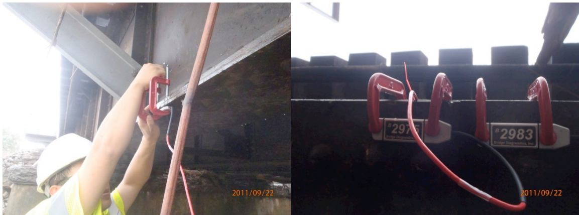
Figure 20. Strain transducers Installation
