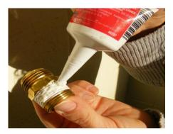
Cover the threads and tape with a layer of sealant. The overflow fitting threads are slightly larger in diameter than the faucet threads, so once you start threading into the barrel by hand, you will quickly need to use an adjustable wrench to tighten the fitting.
