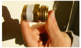
Wrap thread tape around two thirds of the pipe thread side of the garden hose adaptor. The pipe threads are finer then the hose threads. Leave the bottom third of the threads uncovered, similar to the way the faucet was done.
