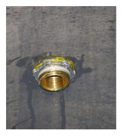
First cover half the threads and around the barrel wall with sealant, then screw the locknut on and tighten down using the groove joint pliers.
