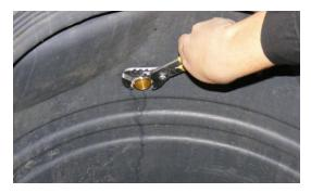
Thread the locknut to the inside threads of the overflow.
