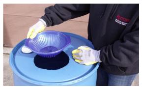
*Inlet:* Use a jig saw to cut an 8-inch diameter hole in top of barrel. Or, if using a pond basket, colander, or other device for the inlet, cut the opening to fit the device without gaps to avoid allowing in mosquitoes.
