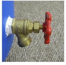
Smooth the excess sealant around the base of the faucet.
