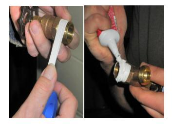
Wrap two thirds of the faucet threads with two layers of the thread seal tape. Leave the bottom third of the threads uncovered so it will be easier to start threading into the barrel. Apply a layer of sealant over top of the tape and threads. Use latex-free gloves when using silicone sealant (caulk).
