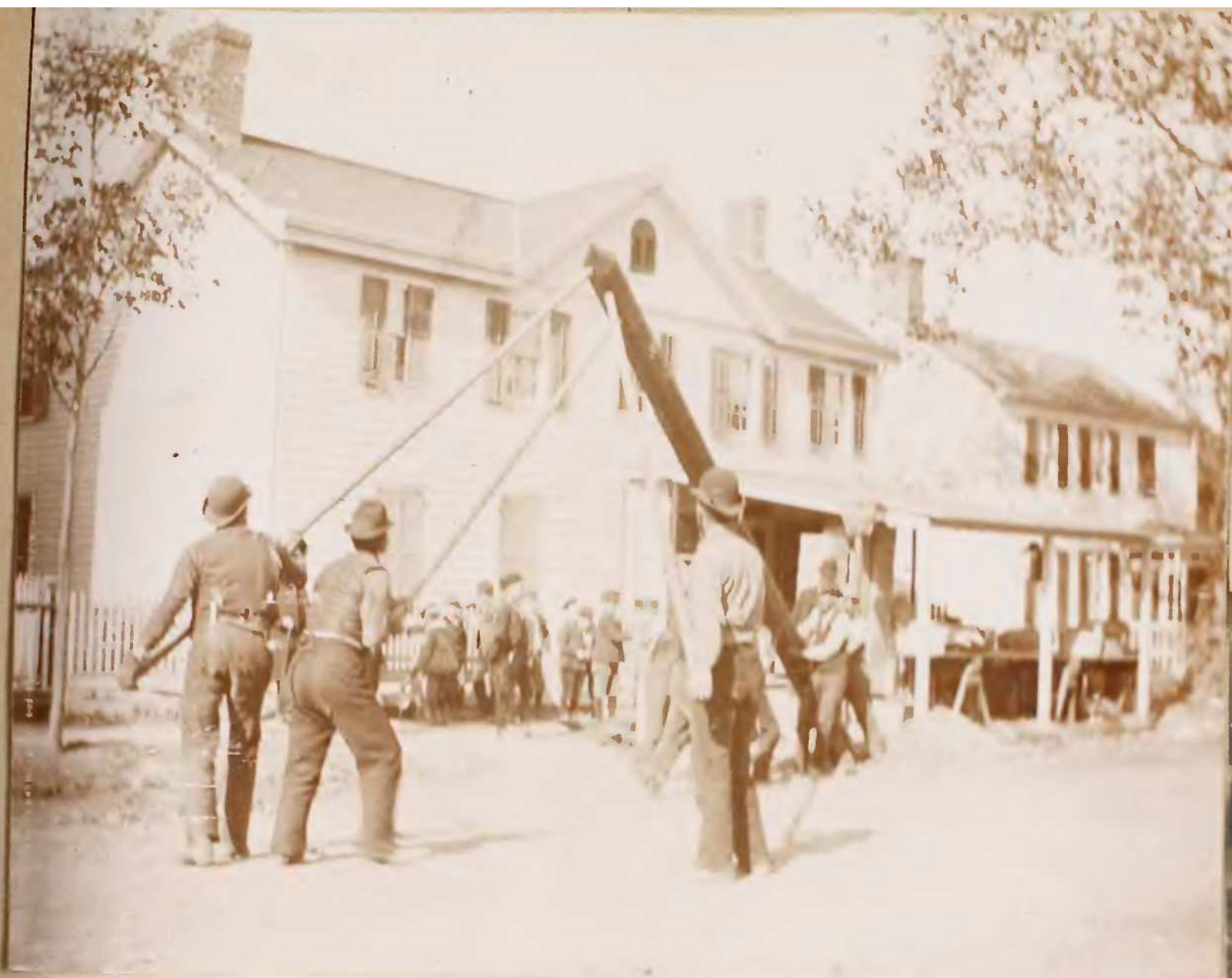
146 Raising Trolley Poles; Main St. opp. J.B. Tuttle's Oct 1895
