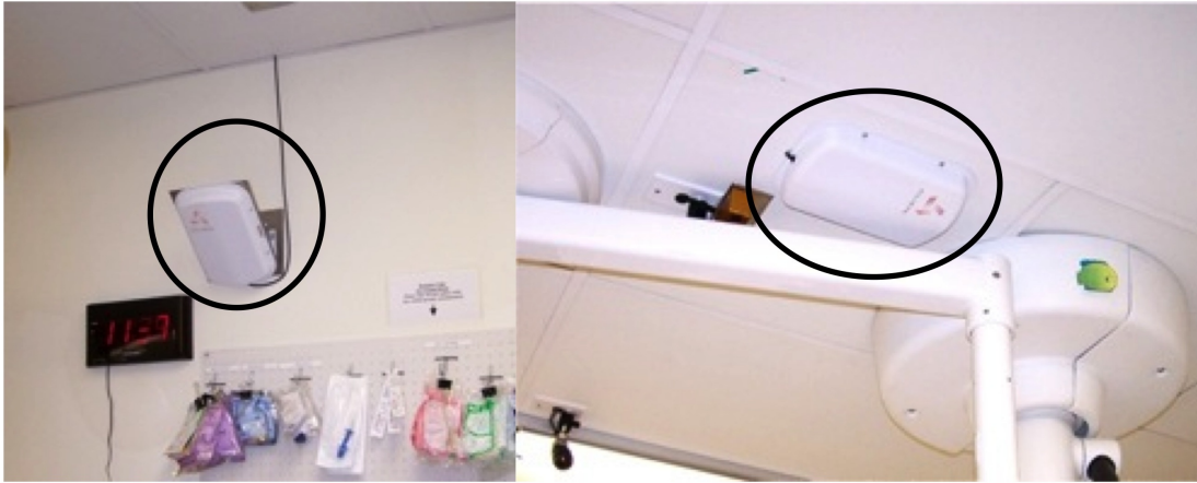
Figure 6.7: Positioning of angled and ceiling-mounted antennas at CNMC. Left picture shows angled antenna #1. Right picture shows ceiling-mounted antenna #3
