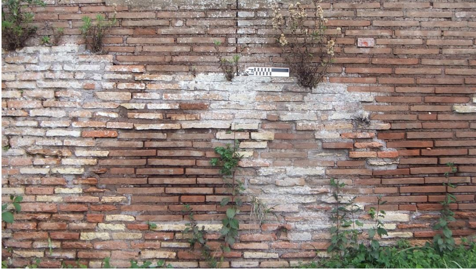
Figure 8: Salt efflorescence in room 97. Note that the modern (1964) brick above, to the right, and left of center is not affected (although the restoration plaque at top right has been). Photo by author.
