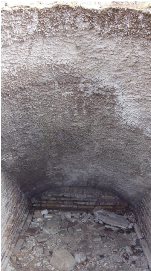
Figure 9: Heavy salt efflorescence in room 92. Photo by author.
