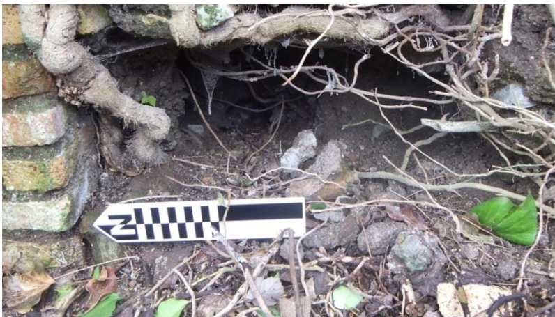
Figure 5: Vegetative damage combined with animal burrowing creates a large lacuna in the southwest wall of room 75. Photo by author.
