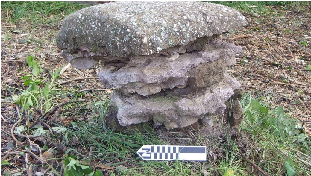
Figure 10: Crumbling pier with too-large concrete cap in room 76. Photo by author.
