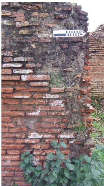
Figure 19: Exposed core in pier in room 82. Photo by author.
