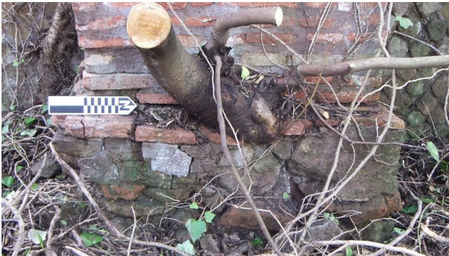
Figure 4: Vegetative damage to a pier in room 75. Photo by author.
