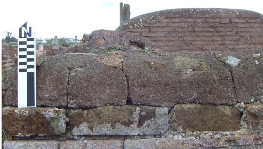
Figure 22: Deteriorating cement wall cap from room 73.
