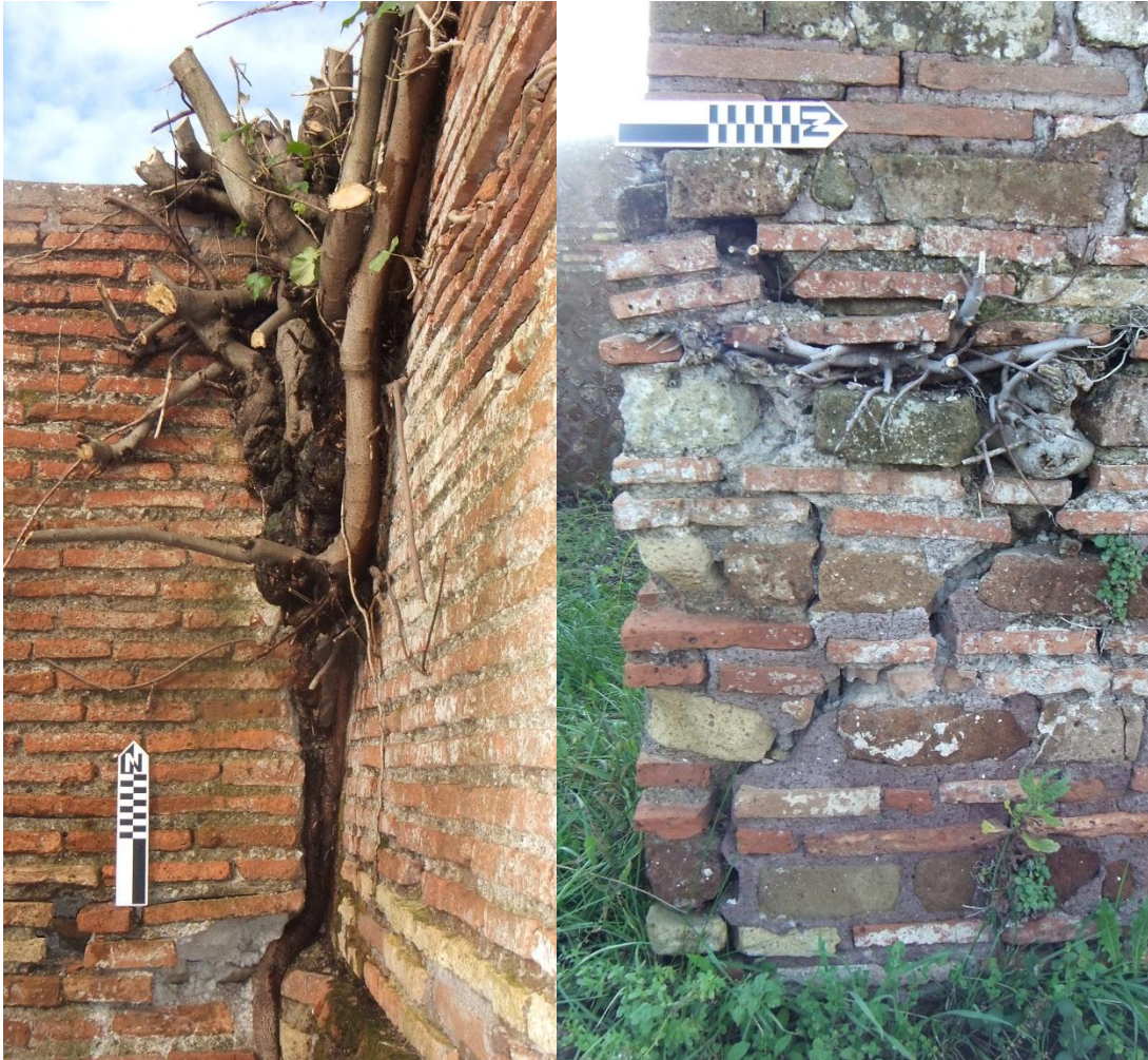
Figure 6: On left, large trunk pushes apart north and east walls in room 79. On right, invasive vegetation tears apart wall in room 68. Photos by author.
