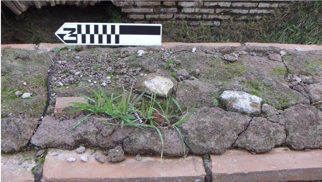
Figure 12: Inadequate concrete capping to wall in room 73, now extremely friable. Photo by author.
