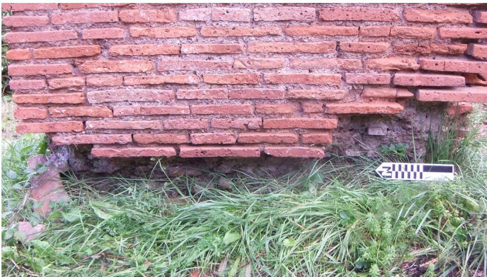
Figure 20: Base of pier in room 85, with substantial loss of brick and mortar at base. Photo by author.
