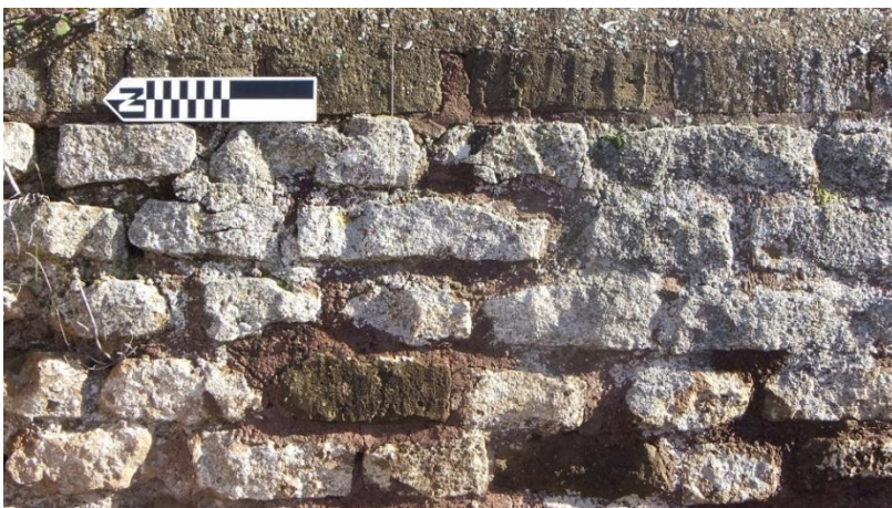
Figure 7: Salt efflorescence on eroded brickwork in room 76. Photo by author.
