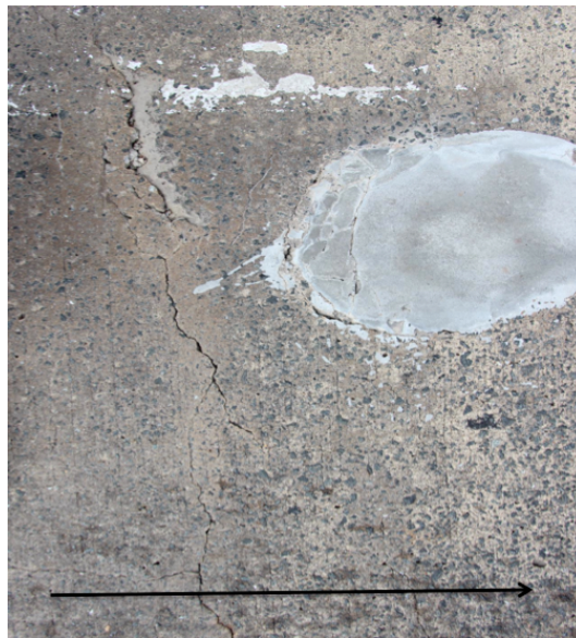
Figure 1.6: Transverse cracks on the surface. The black arrow indicates the direction of travel of the robot during image collection.
