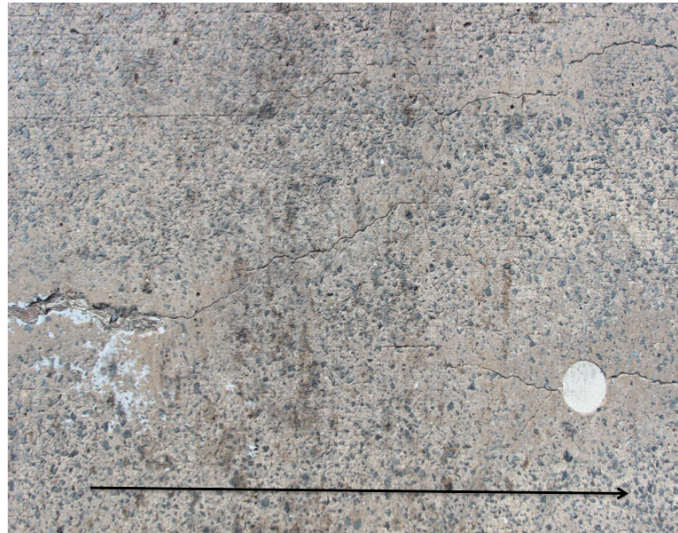
Figure 1.8: Cracks along various directions. Known as pattern or map cracks. The black arrow indicates the direction of travel of the robot during image collection.
