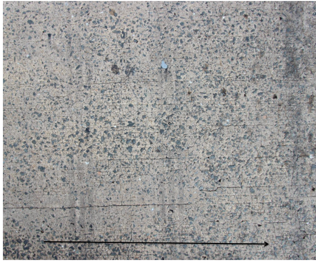
Figure 1.7: Longitudinal cracks on the surface. The black arrow indicates the direction of travel of the robot during image collection.
