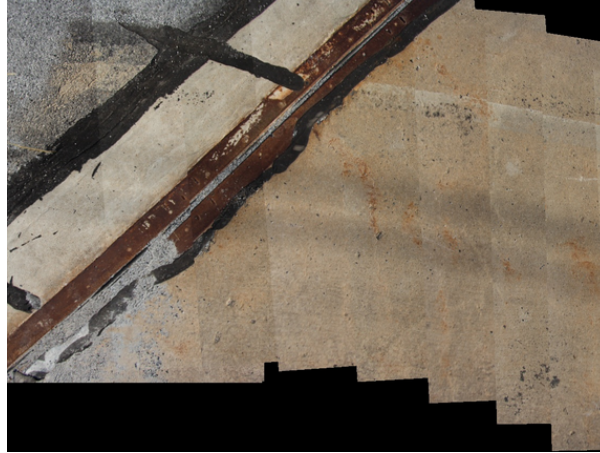
Figure 5.4: Improper stitching due to reprojection and distortion error.
