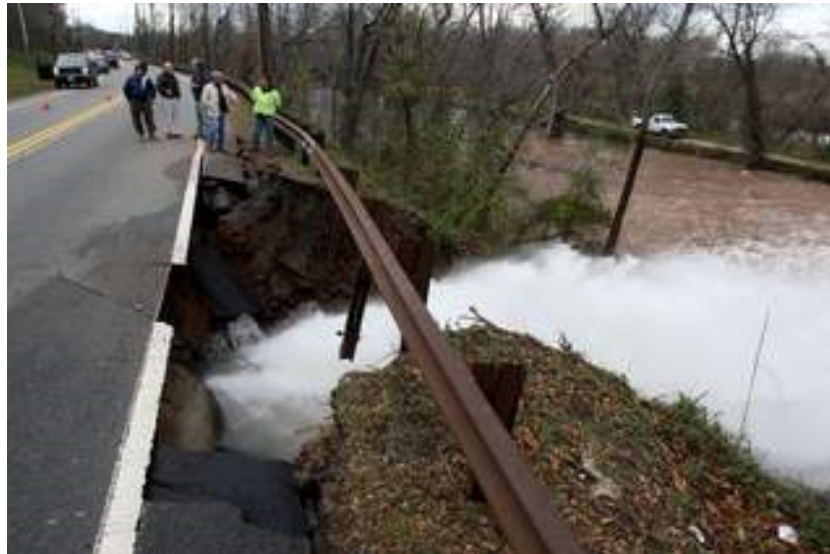
Sixty inch water main break on Weston Canal Road in Franklin
