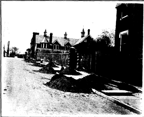
Showing the Rock taken out and the Soil put in
