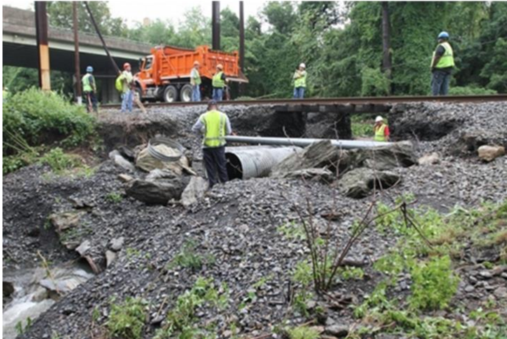
Figure. 5.15 Jenkintown Township, Pennsylvania rail track washout
