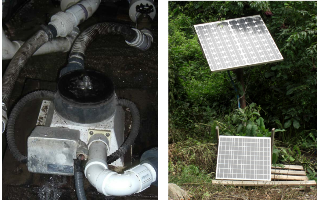
Figure 3.2-A Earthaven micro-hydro turbine and photovoltaic panel photographs
