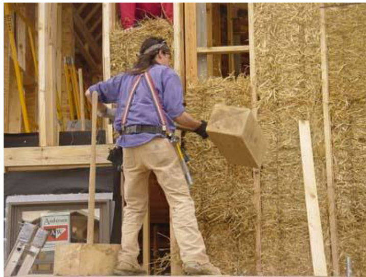
Figure 4.2-D Construction of a home in SONG using straw bale techniques 9
