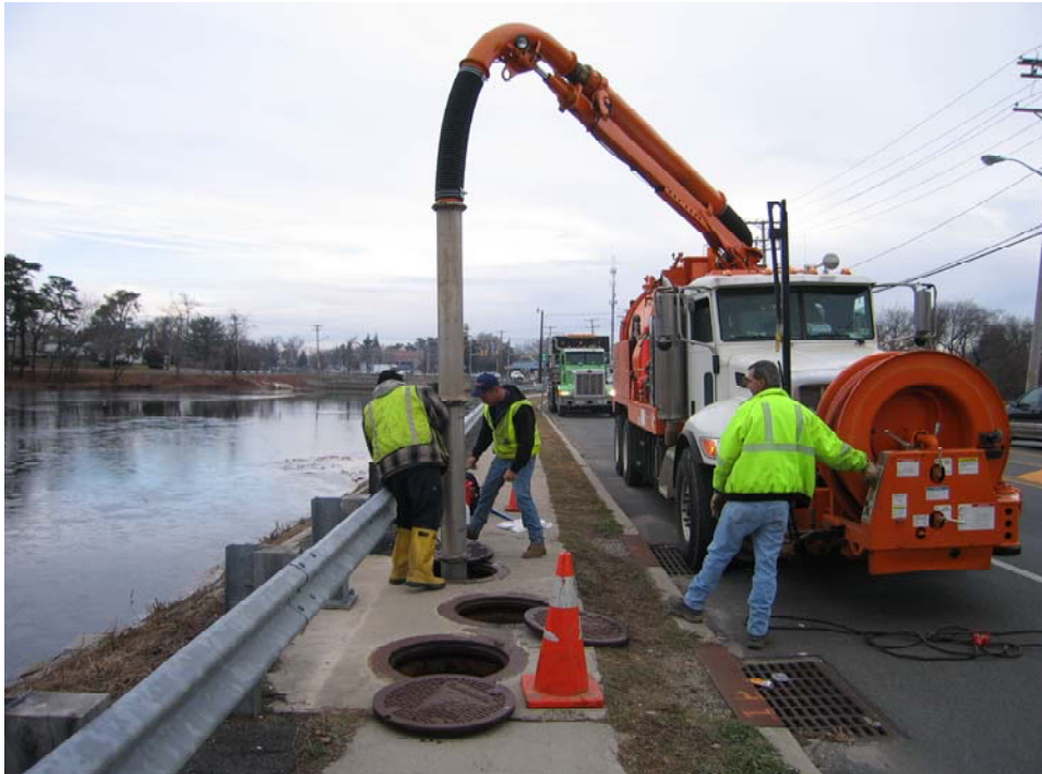
Figure 4.2 Pump out water first and then pump out solids (Typically)
