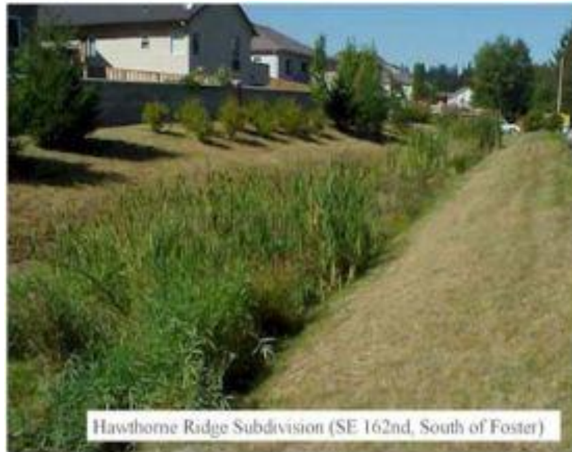
Figure 6. Image showing an installed swale (Source – ecosrq.com)
