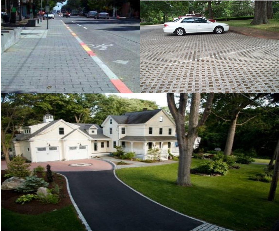
Figure 9. Permeable sidewalk-source-naturalpathlandscaping.com(Top left); Figure 10. Permeable parking-source-ralieghnc.com(Top right); Figure 11. Permeable driveway-source-dailysightline.com(Bottom)
