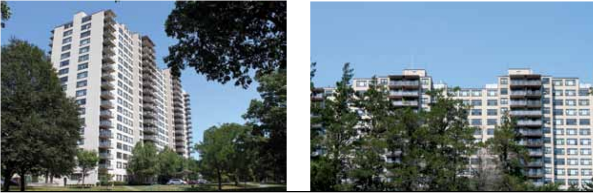
FIGURE 7. Views of a high-rise luxury apartment complex in New Brunswick, New Jersey, constructed in the early 1960s.
