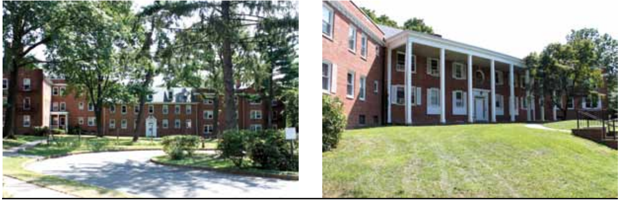
FIGURE 6. Views of a garden apartment complex in Highland Park, New Jersey, built in the late 1940s.
