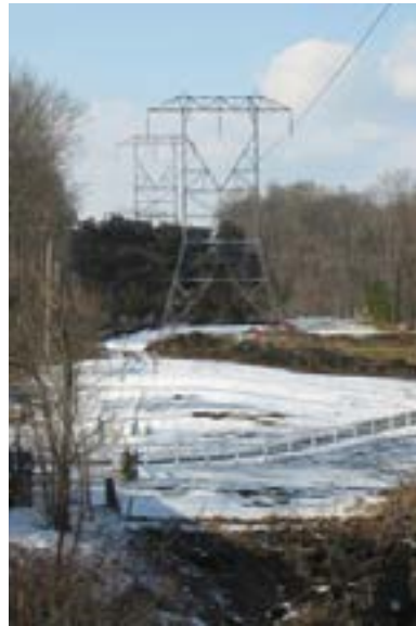
A lattice tower on the permanently preserved Pattison farm in Andover Township, Sussex County, is being replaced as part of PSE&G's Susquehanna-Roseland electrical transmission upgrade project.
