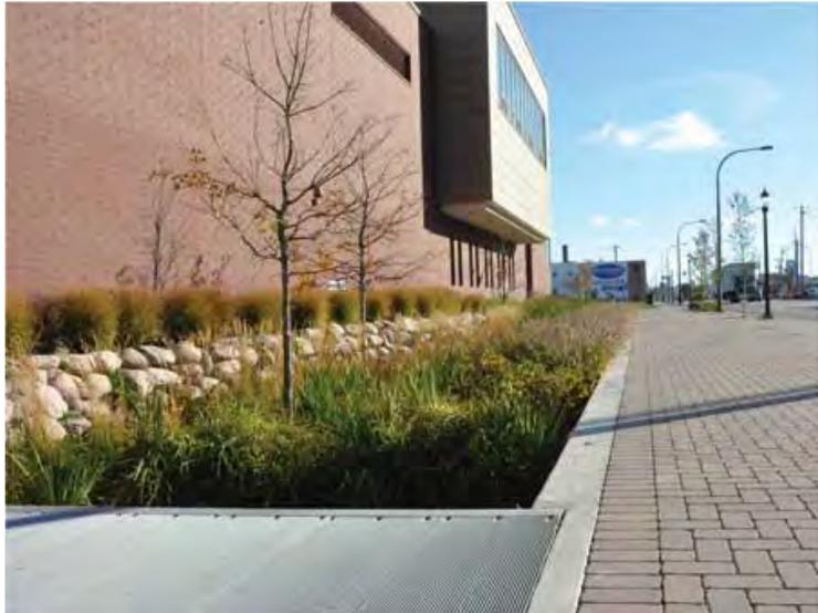
**Figure 1-1:** Bioswale, Chicago, Illinois. (CE News, [www.cenews.com/article/8895/turning\\_stormwater\\_into\\_a\\_resource](http://www.cenews.com/article/8895/turning_stormwater_into_a_resource))
