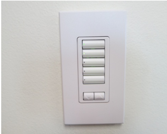
Figure 26. Intuitive? Example of a Lighting Control that does not Provide Clear Direction to its User. Source: Rutgers Center for Green Building Photo Archive.
