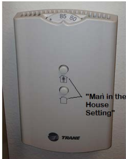
Figure 11. On/off “Man in the House Thermostat Type.
