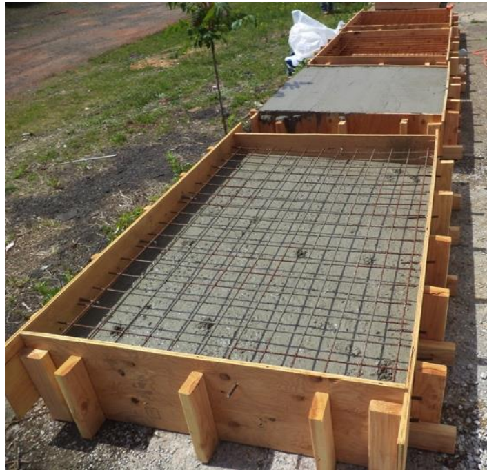
Figure 7.3 Casting Process - Day 1
