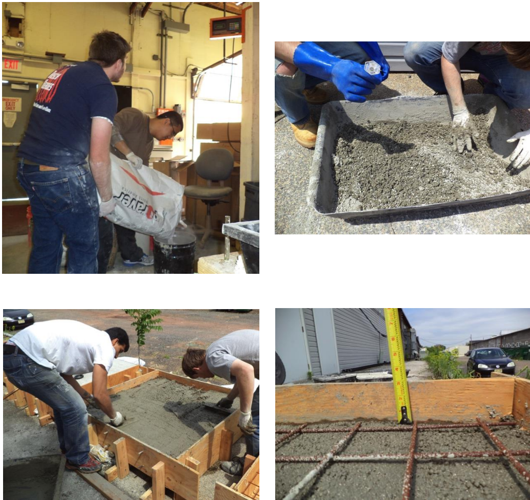
Figure 7.5 Light weight concrete mixing procedure-Day 2
