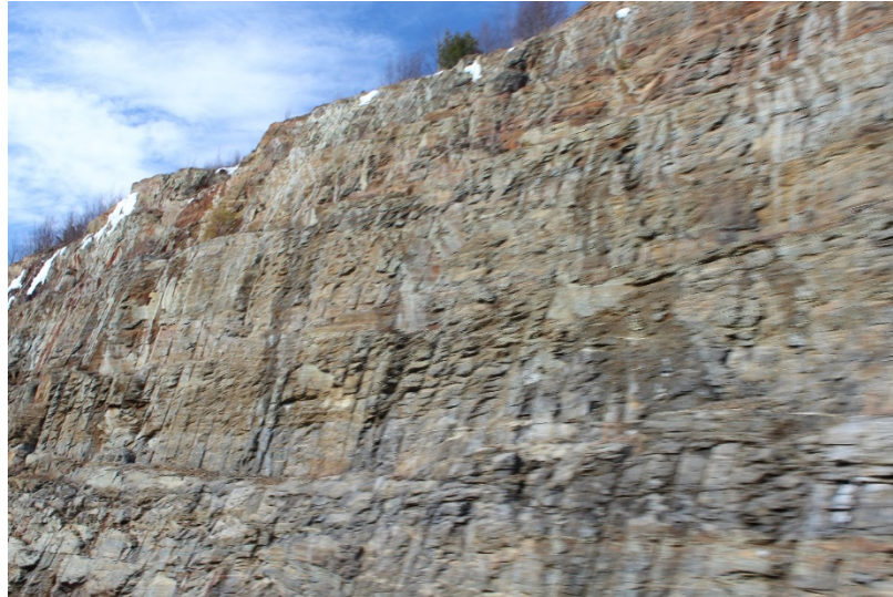
Figure 6.19: Vertical Dynamite Drill Lines along I-40
