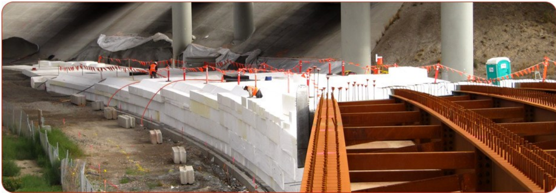
Figure 8: EPS Geofoam Being Used as Abutment Backfill (Geofoam Applications and Uses)
