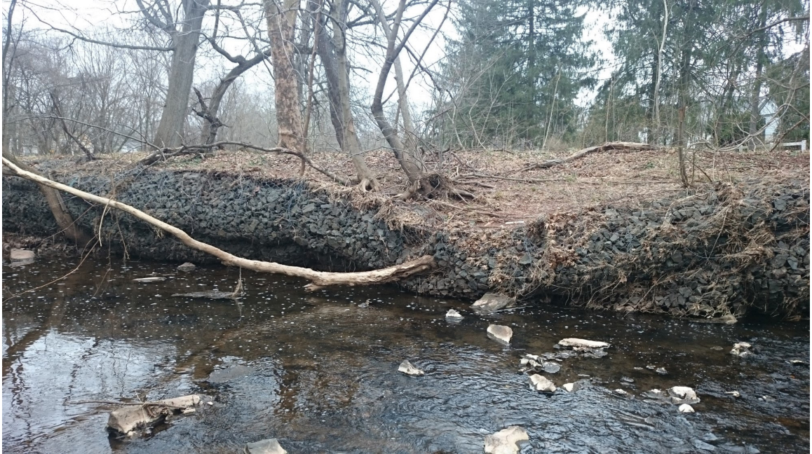
Figure 14. Existing gabion wall beginning to fail.
