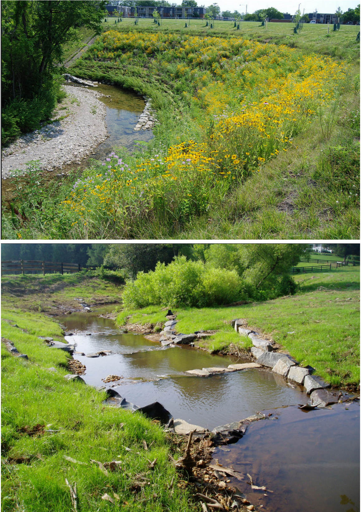
Figure 40. Beaver Run case study strategies. From top: Terrace Walls, Plunge Pool. (Images: Mill Creek Watershed Council)
