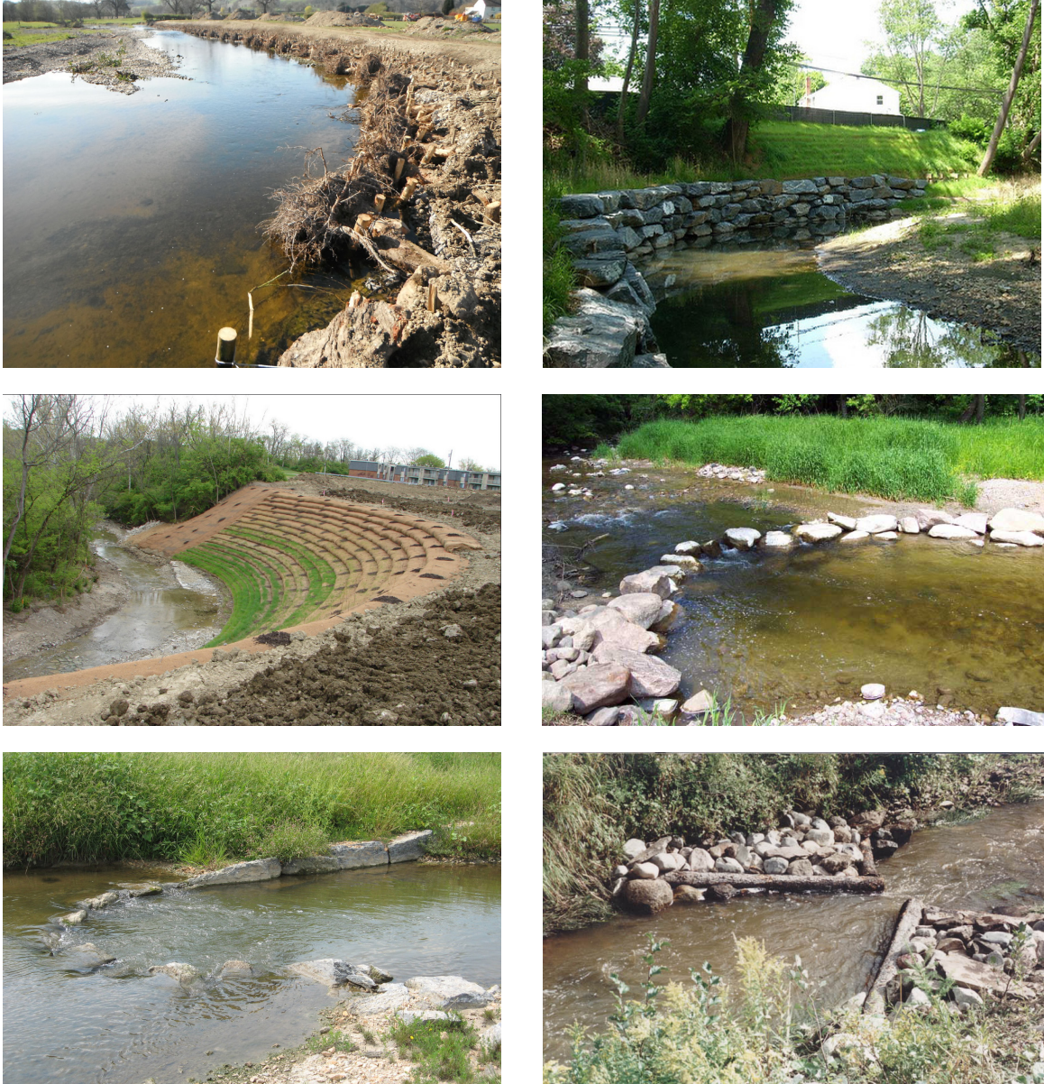
Figure 41. Best Management Practices strategies. From top left: Rootwad Revetment, Stacked Stone, Natural Fiber Matting, Rock Cross Vane, J-Hook Vane, Wing Deflectors. (Images: Salix River Restoration Specialists, Montgomery County, Maryland DEP, Mill Creek Watershed Council, Minnesota River Basin Data Center, Aquatic Resource Restoration Company, New Mexico State Forestry)
