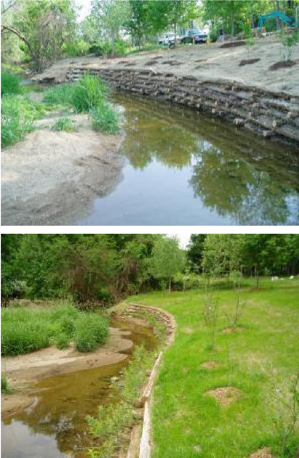
Figure 37. Peapack Brook case study strategies. From top: Live Cribwall, Native Riparian Planting via live stakes. (Images: Amy S. Greene Environmental Consultants, Inc.)
