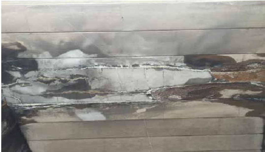
Figure 7.1 - Damaged Beams BM3 and BM 4 in Span 1
