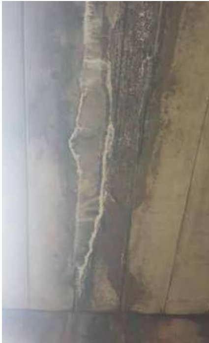
Figure 7.3 - Damaged Beams BM3 and BM4 in Span 4
