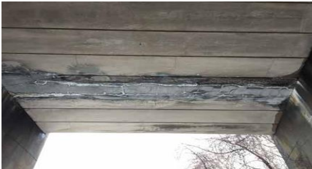
Figure 7.2 - Damaged Beams BM18 and BM19 in Span 1
