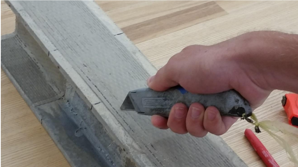
Figure 45: Using a knife to cut the basalt fiber on bottom flange
