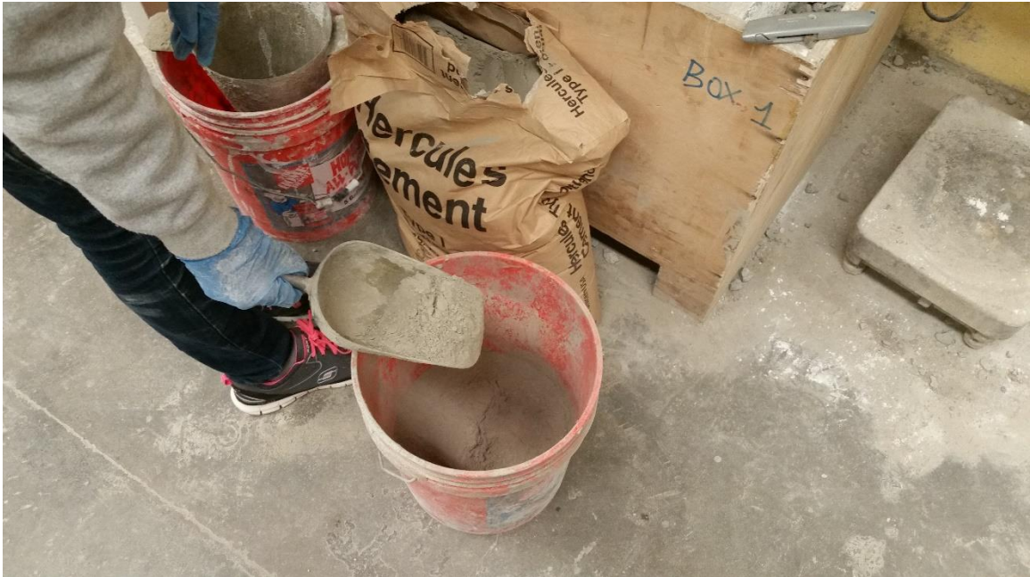
Figure 2: Batching cement
