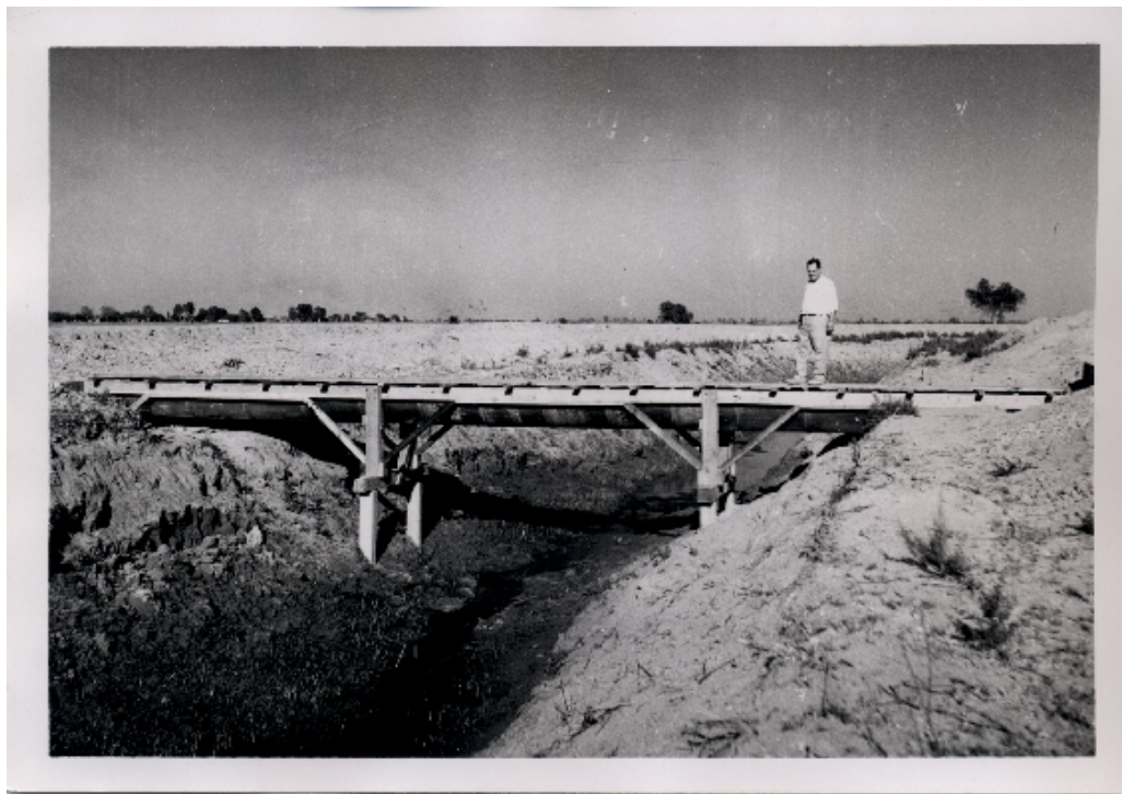
A deteriorating drainage ditch, which is eroding and filling with silt. Such a ditch can only lower the water a few feet in the adjacent areas. Many parts of the region lacked even this form of drainage infrastructure. Source: Archivo Histórico del Agua, Colección Fotográfica.
