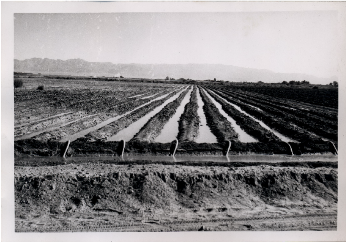
Flood irrigation under way in Mexicali. The tubes siphon water into the plot from the canal in the foreground, flooding each furrow. Enormous volumes of water are lost to evaporation with this method. Source: Archivo Histórico del Agua, Colección Fotográfica.
