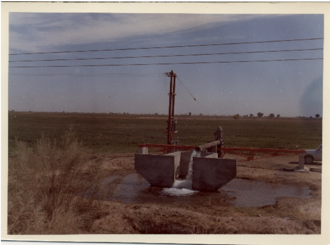
A well constructed by the Secretaría de Recursos Hidráulicos in the Mexicali Valley. SRH-operated public and cotton industry-financed private wells multiplied in number as the volume and quality of surface water diminished from 1955 onwards, with deleterious effects on Mexicali's aquifer. Source: Archivo Histórico del Agua, Colección Fotográfica.
