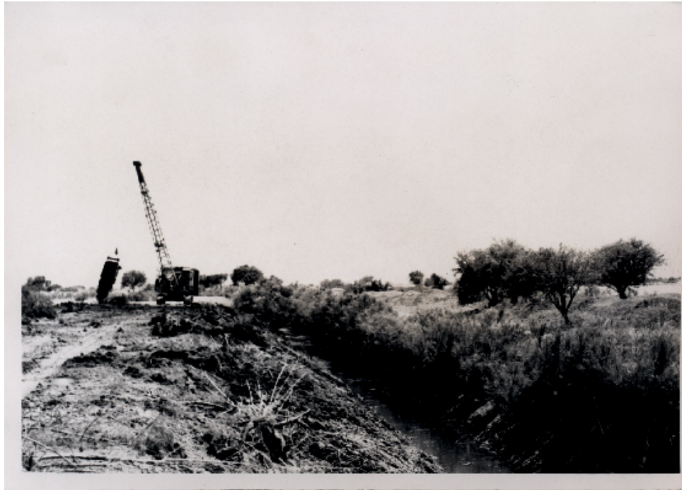
An irrigation canal overgrown with vegetation, which causes water loss through transpiration and reduces the canal's volume and efficiency. The machinery at left is part of an effort to clear canals of vegetation. Source: Archivo Histórico del Agua, Colección Fotográfica.
