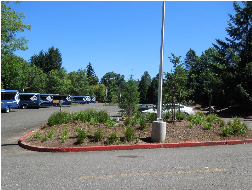
Figure 64: Raingarden retrofitted into the end island. Photo by author.
