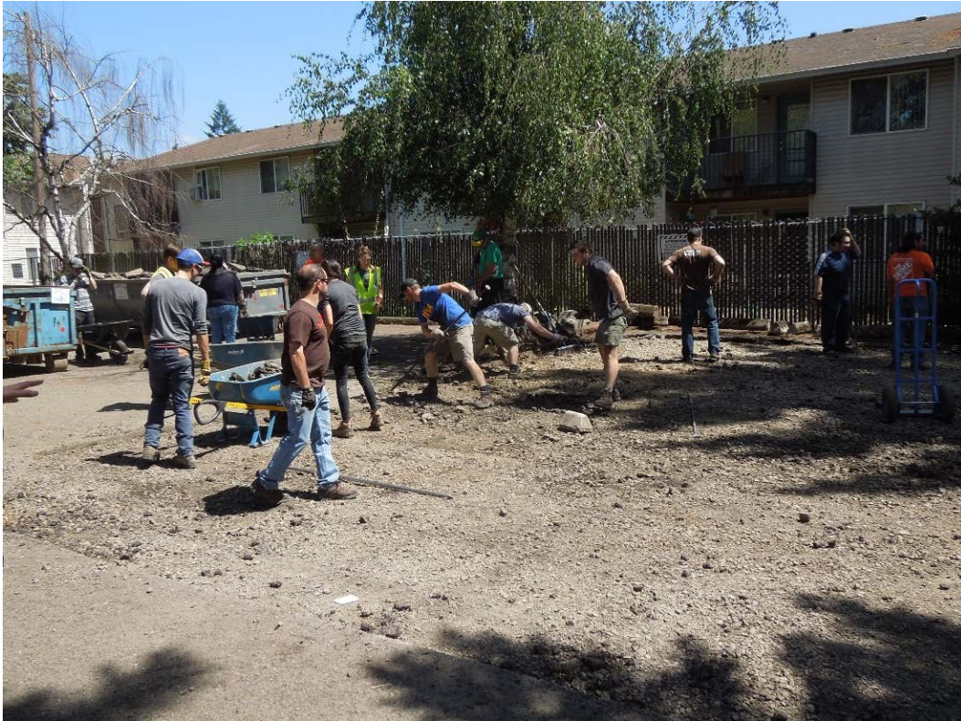
Figure 66: Removing the final pieces of asphalt. Photo by author.
