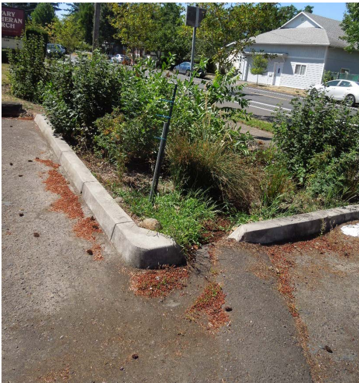
Figure 68: A speed bump, bottom right, channels water to a rain garden. Photo by author.
