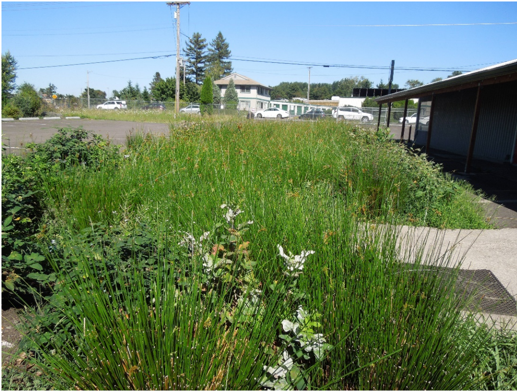
Figure 70: A large raingarden planted in removed asphalt mitigated flooding at St. Mary's Ethiopian Church, Portland. Photo by author.
