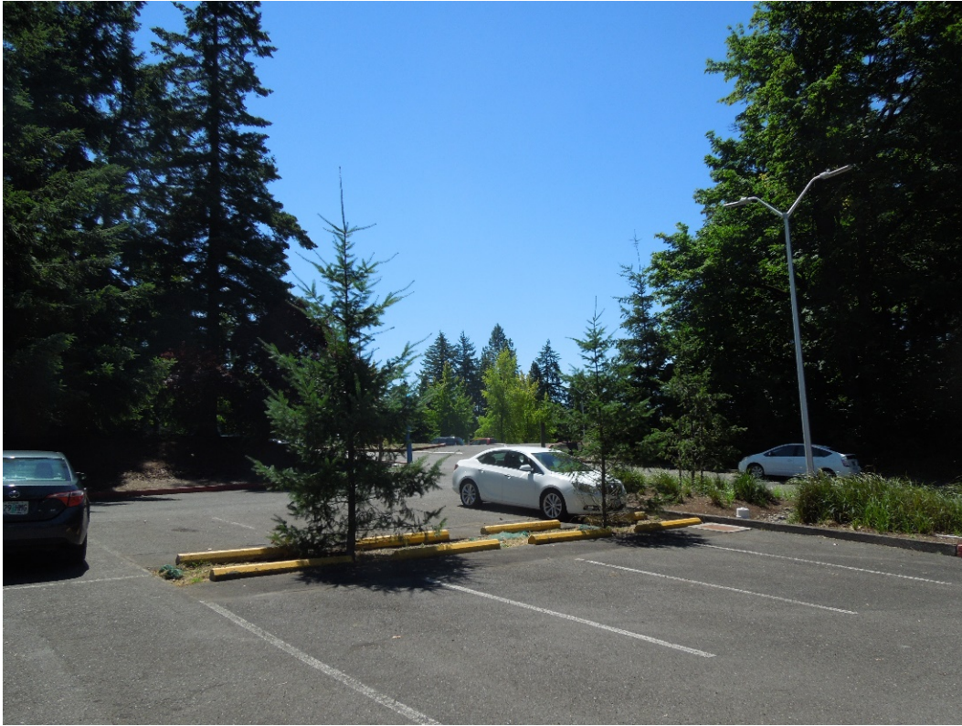
Figure 63: Portland Community College demonstration of porous asphalt, structural soil and small planting pits. Depave volunteers removed the asphalt for this project. Photo by author.
