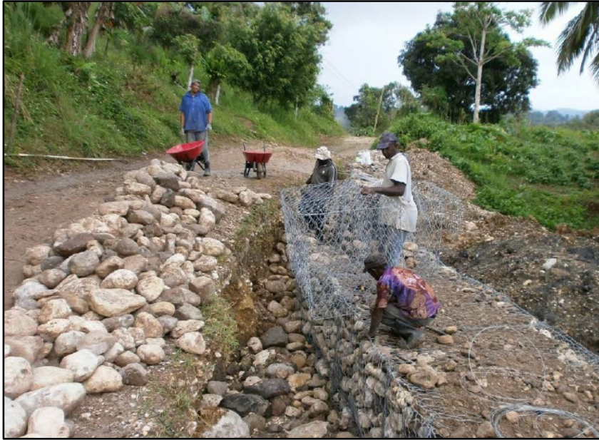
Figure 22. Jeffrey Town community members constructing gabion baskets to reduce landslides. (Credit: JTFA)
