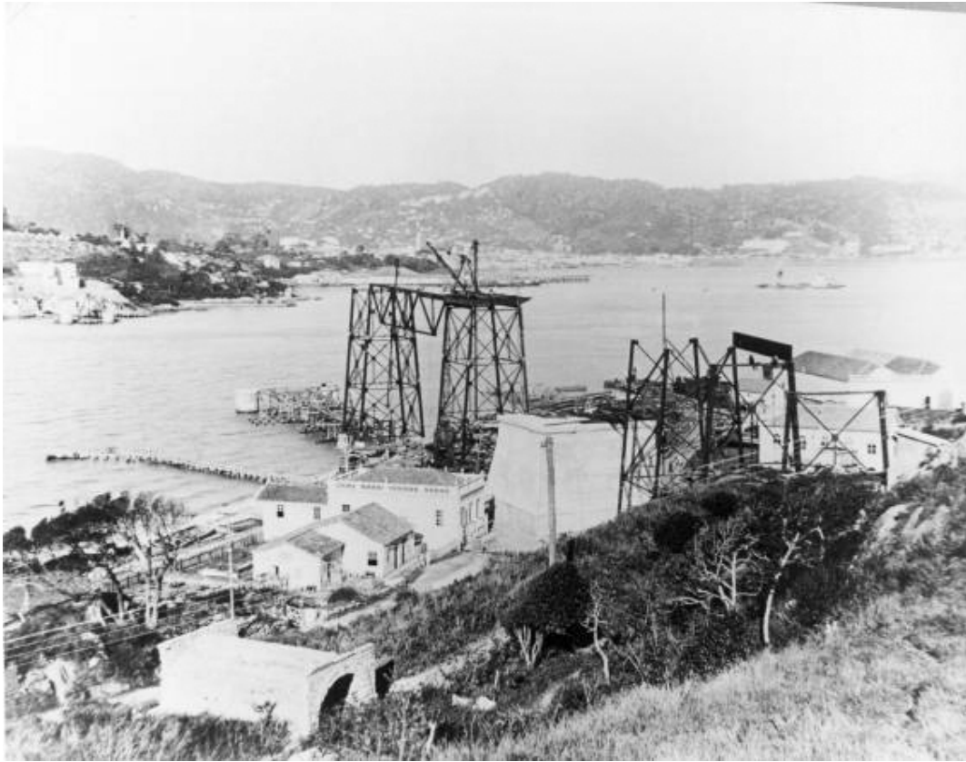
Figure 8. Construction of the Point Hercílio Luz suspension bridge, 1920-1926.
