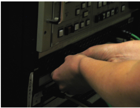
Figure 7 – Patching Cables in Patch Bay (Digital Photos Taken by Author at Site L2)
