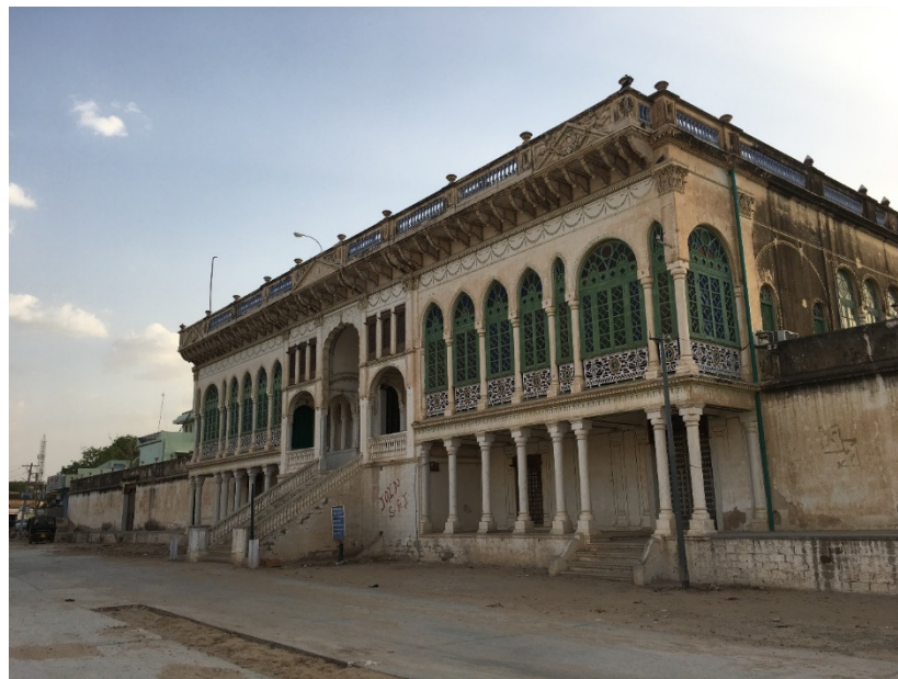
Figure 10. The front facade of the Bhartia Haveli in Fatehpur-Shekhawati relies heavily on Belgian glass for decoration. The prevalence of openings on the front facade allow for ventilation. Source: Author Image
