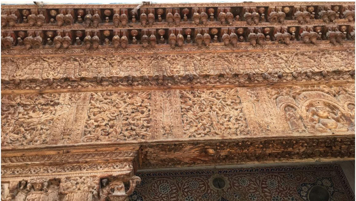
Figure 18. The teak wood beam seen at the entry way of the Nadine le Prince Haveli. The carving was quite elaborate, and the wood shows no wear though it has been exposed to the elements for 200 years. Source: Author Image
