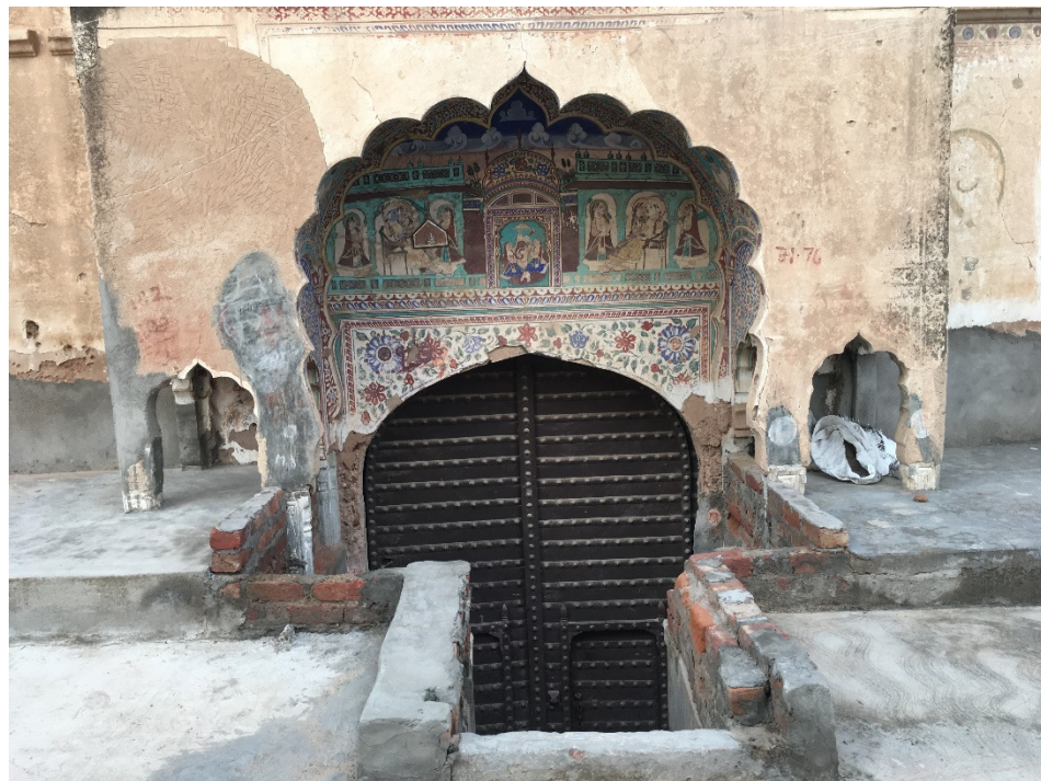
Figure 20. The concrete wall used here demonstrates the damage in the Fatehpur-Shekhawati havelis . The frame of the door is already crumbling and in some instances the concrete has chipped off revealing the mortar. Source: Author Image
