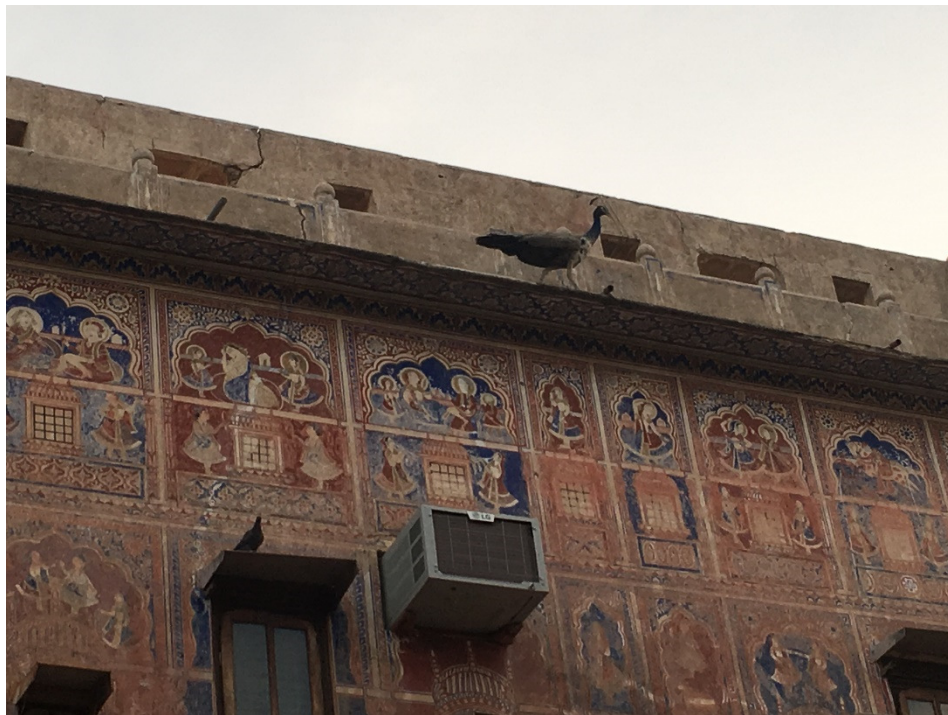
Figure 30. The red pigment, which was not adhered properly during the restoration of the exterior façade of the Nadine le Prince Haveli, bled down the walls following monsoon rains giving the façade the red tinge. Source: Author Image
