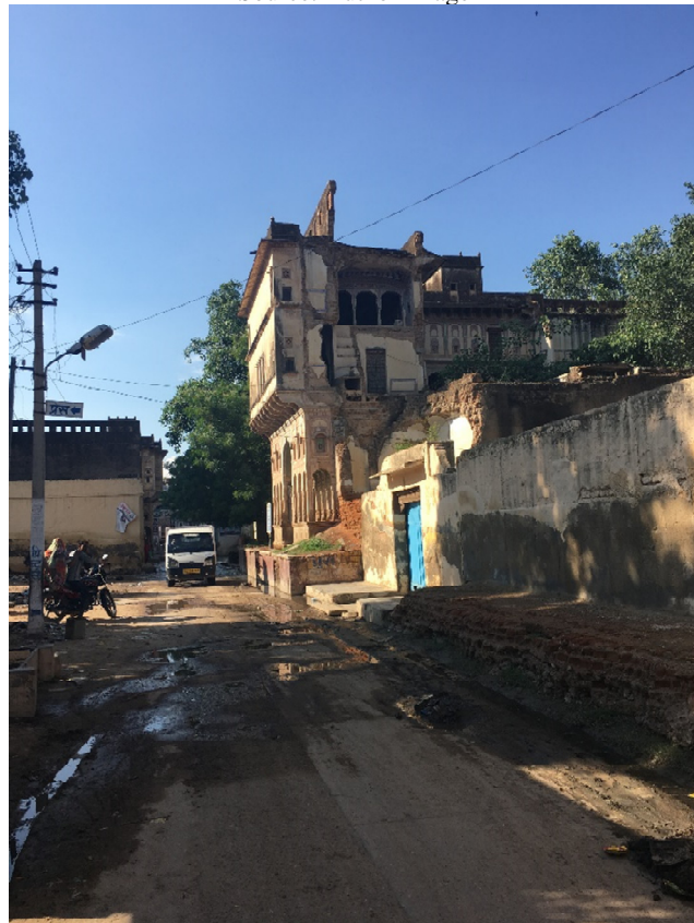
Figure 38. Haveli , in Fatehpur-Shekhawati, whose one side has sheared off. If there is any further structural damage, the haveli will fall. Source: Author Image
