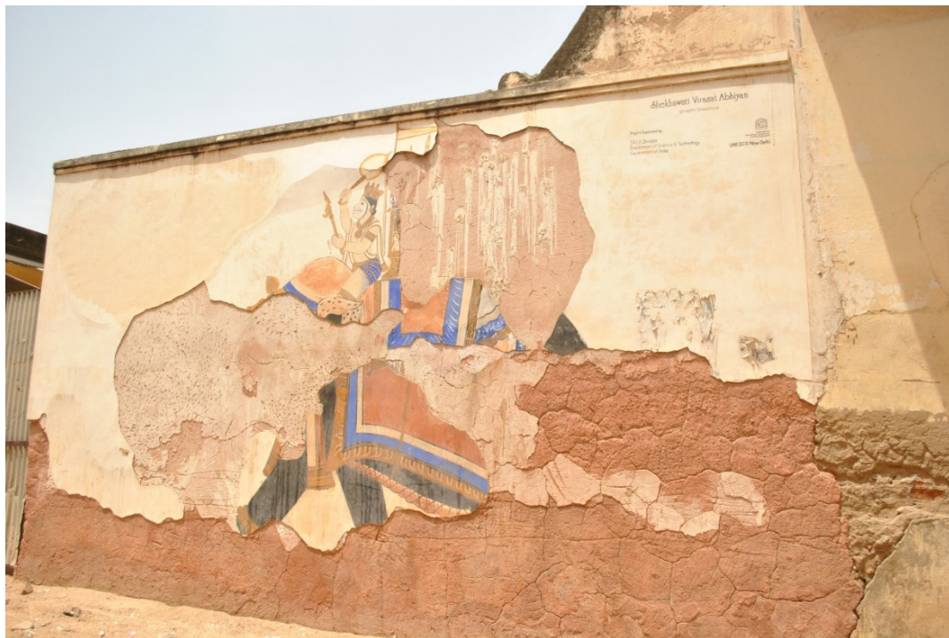
Figure 22. The elephant fresco put up by UNESCO's New Delhi Office and INTACH's Shekhawati Chapter. The fresco has chipped off because there was poor adherence in the plaster layers and water damage that was creeping up from the bottom of the wall. Source: Author Image
