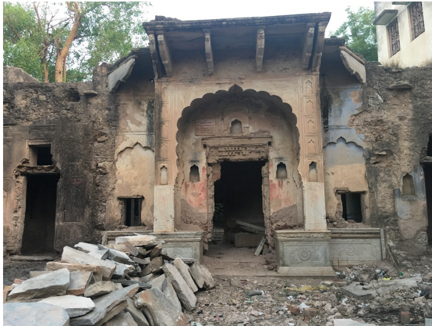
Figure 37. Another abandoned haveli , in Fatehpur-Shekhawati. All the wooden pieces are no longer present and the stone lying around will be salvaged as building material as well.
