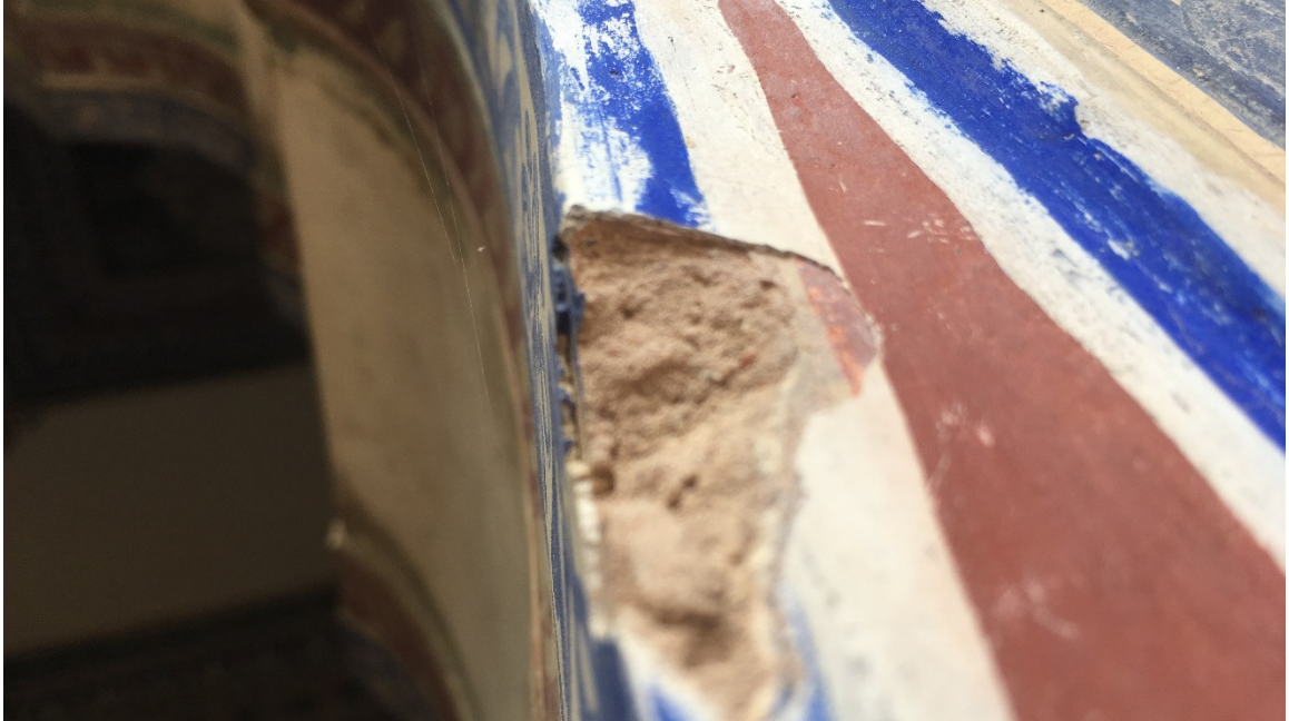
Figure 15. The plaster for the fresco was layered in thin portions and painted while wet. The red pigment has seeped through the layers of plaster and onto the mortar below. Additionally, it does not have the texture of the mortar.
