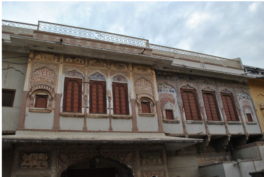
Figure 6. Frescoed exterior façade. Some of the frescoes have faded and some have been covered up with acrylic paint. Source: Author Image
