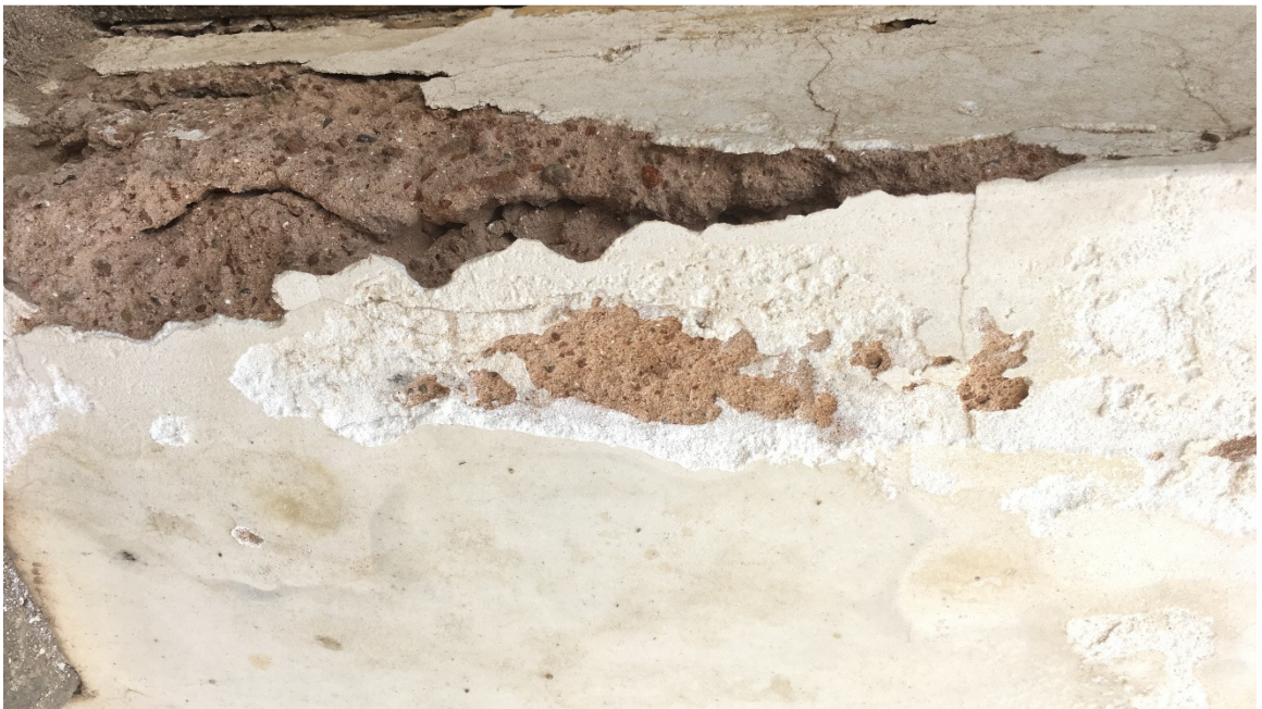
Figure 14. The dhandhala was also mixed into this mortar. The lower-right hand corner shows use of more-modern limestone, which is bright white. Source: Author Image
