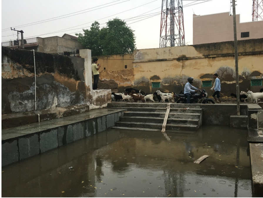
Figure 41. The barrier situated in front of the Nadine le Prince Haveli. The white pipe will drain out all the water to the street and the drainage system. The image was taken on June 27, 2017, prior to the heavy flooding at the end of the following month. Source: Author Image
