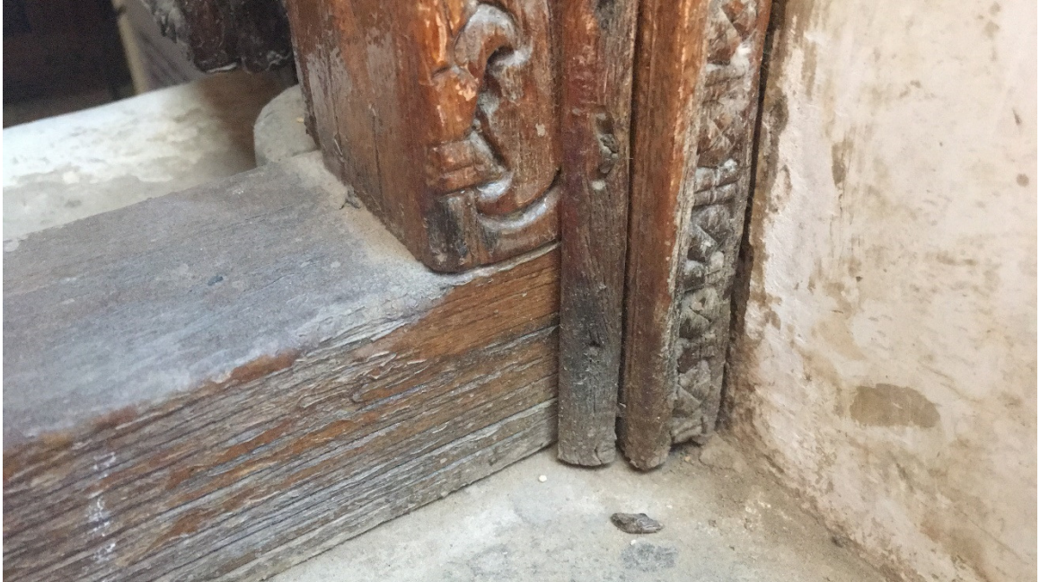
Figure 17. The rohira wood as used in the window frame. The weathering is there in wood, as the wood is original to the Nadine le Prince Haveli. Source: Author Image
