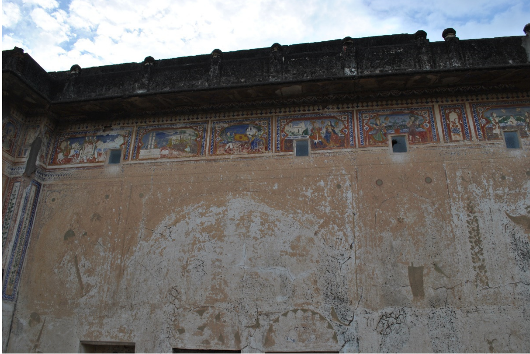
Figure 27. The frescoes of the Bansidar Bhagat Haveli, in Nawalgarh, have faded, but no attempts have been made to preserve them. There is no restoration or conservation work. The top-panel below the overhang is in better condition as it is protected from the elements. Source: Author Image
