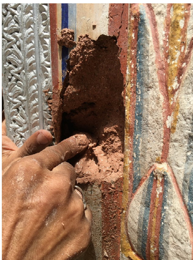
Figure 34. Swarnkar filling in mortar into a part of the wall which had cracked. Most of his repairs were at this scale. Source: Author Image
