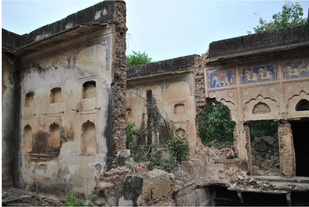
Figure 19. An abandoned haveli . Over the years the damage has exceeded to the point that vegetation has also participated in weakening the structure. Source: Author Image
