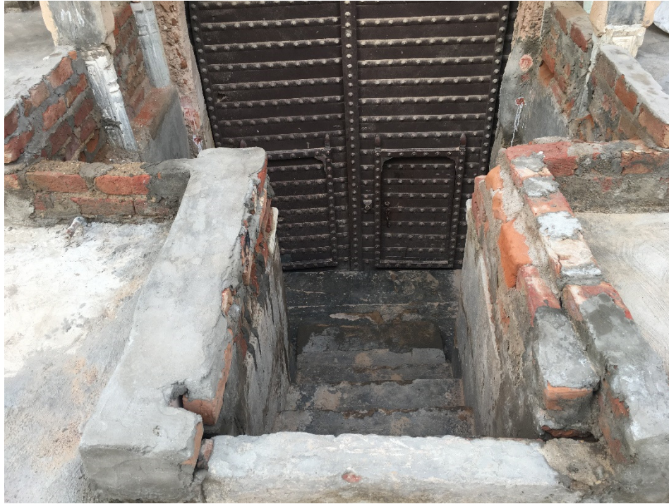
Figure 39. A brick wall built around one of the doors to the house of the Sharma family. The solution is not shocking as much as the difference in street level outside the haveli and ground-level at the bottom of the door. Source: Author Image
