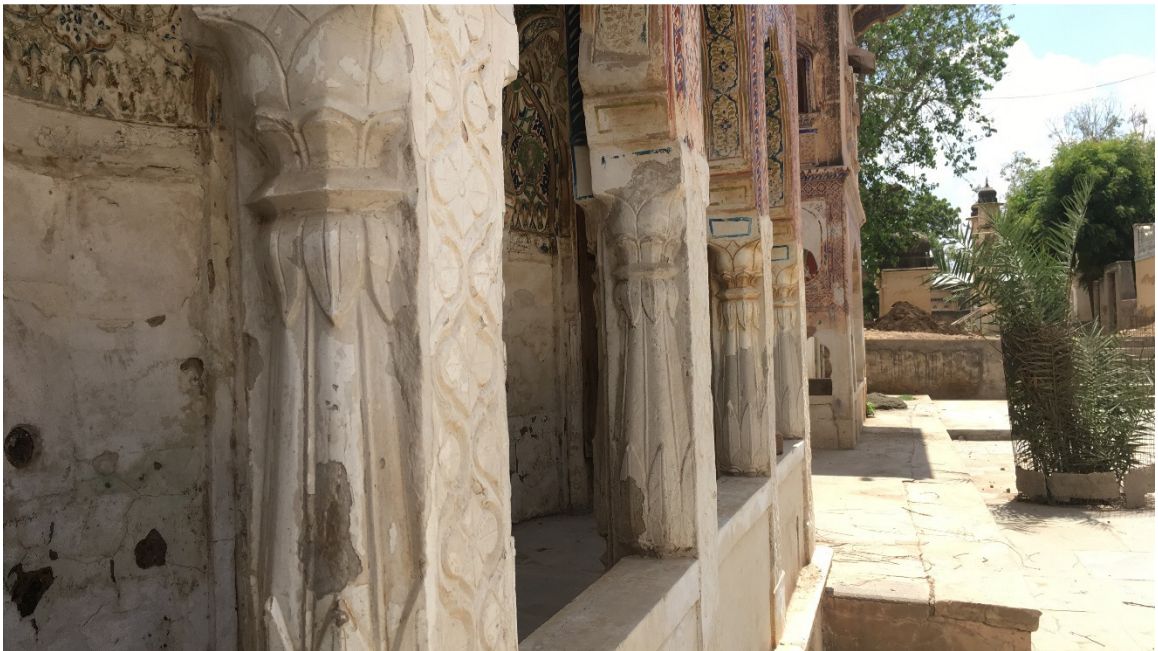
Figure 16. The stone-carved elements at the Nadine le Prince Haveli. They have been covered with plaster to ensure the surface was smooth. In this instance the stone-carved elements serve a structural function. Source: Author Image
