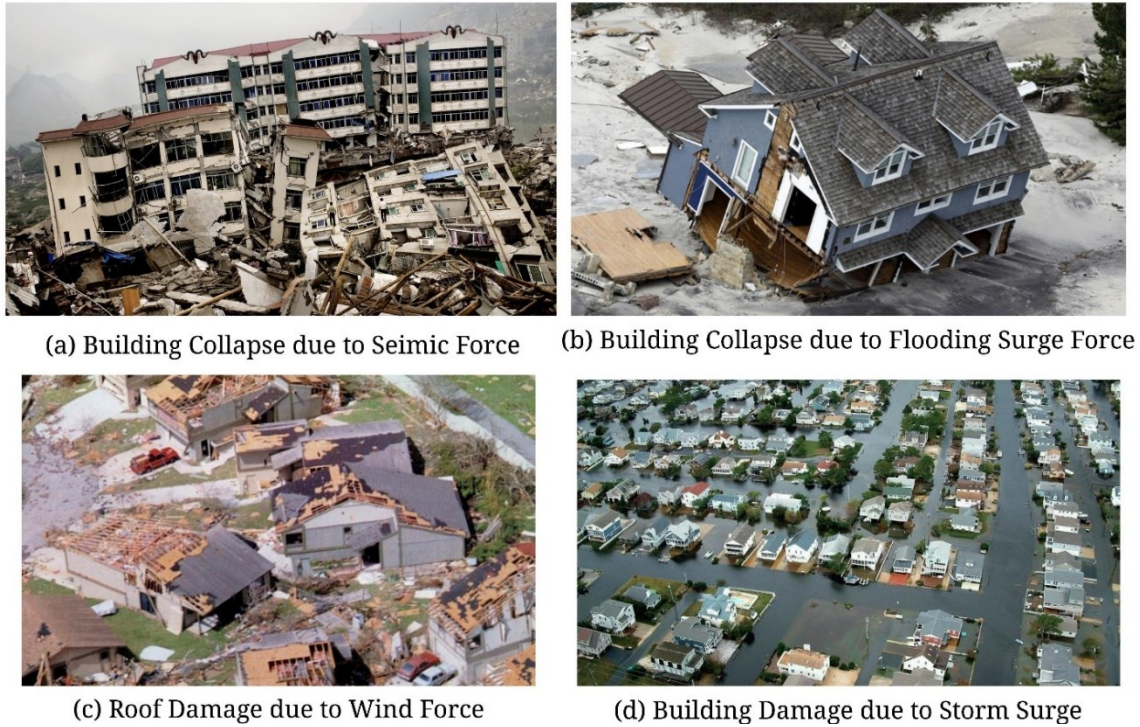
Figure 1.2. Pattern of Seismic-induced and Flooding Surge-induced Building Damage.
