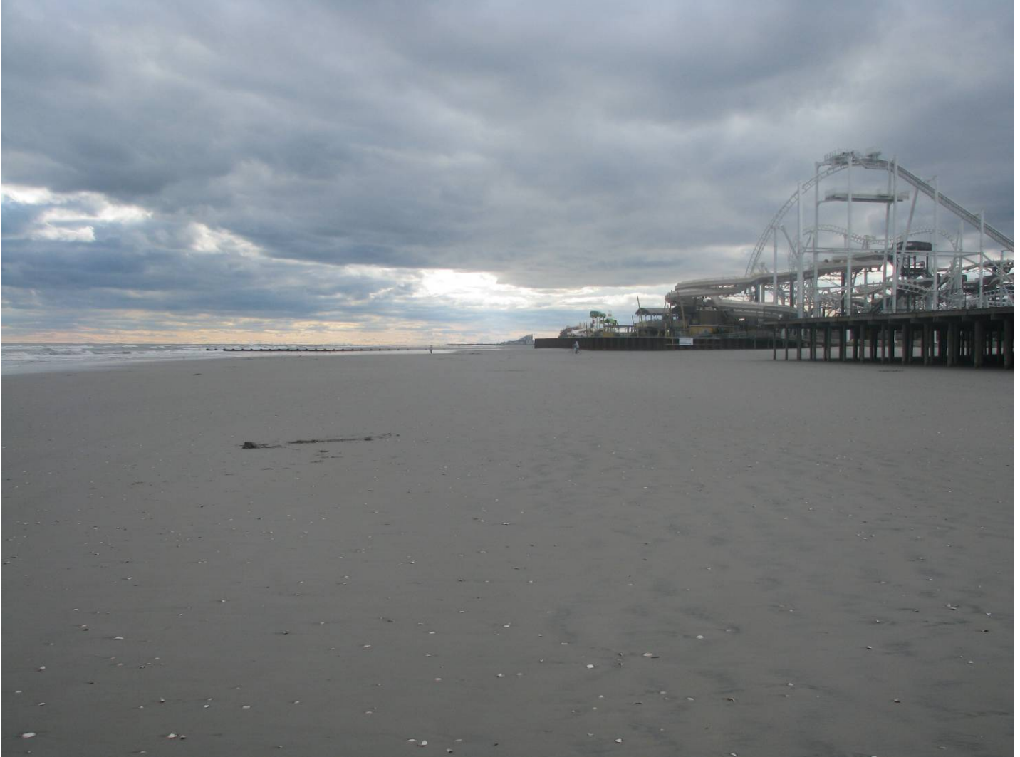
Figure 15. View to the south from 24 th Avenue showing the piers (Morey's Surfside is in the distance) with no remnant of a dune and a very wide intertidal beach seaward of the pier ends. Since Sandy, the beach has accumulated a berm, but the steel bulkhead remains the primary defense for Surfside Pier.
