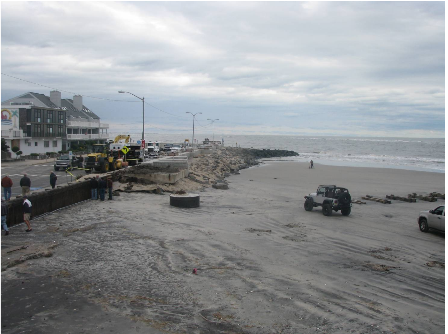
Figure 6. View to the north along the dune line toward the inlet November 1, 2012 immediately following Hurricane Sandy. The gazebo's foundation is to the right of the yellow vehicles on the concrete rubble revetment and the timber bulkhead is exposed on the wet beach. There had been a dune and dry sand beach here prior to the storm.
