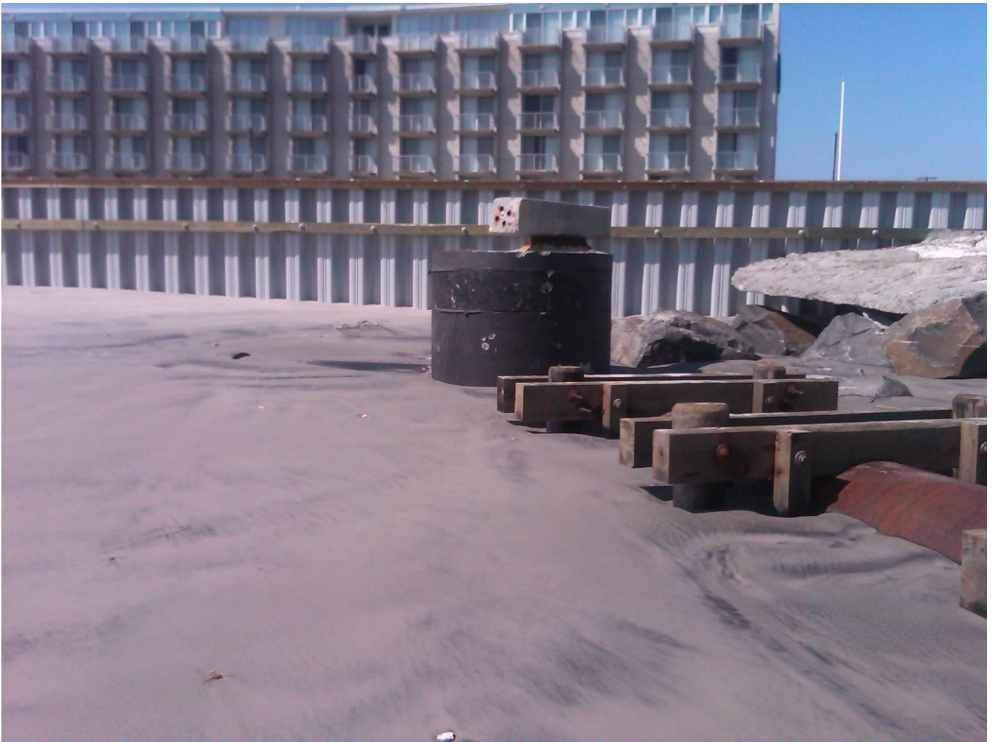
Figure 7. View of the new bulkhead following the March 6, 2013 northeast storm showing the sand loss at the site when compared to the photograph above. Approximately three additional feet of sand has been removed from this location since Hurricane Sandy. This damage was done during the March 6, 2013 northeast storm.
