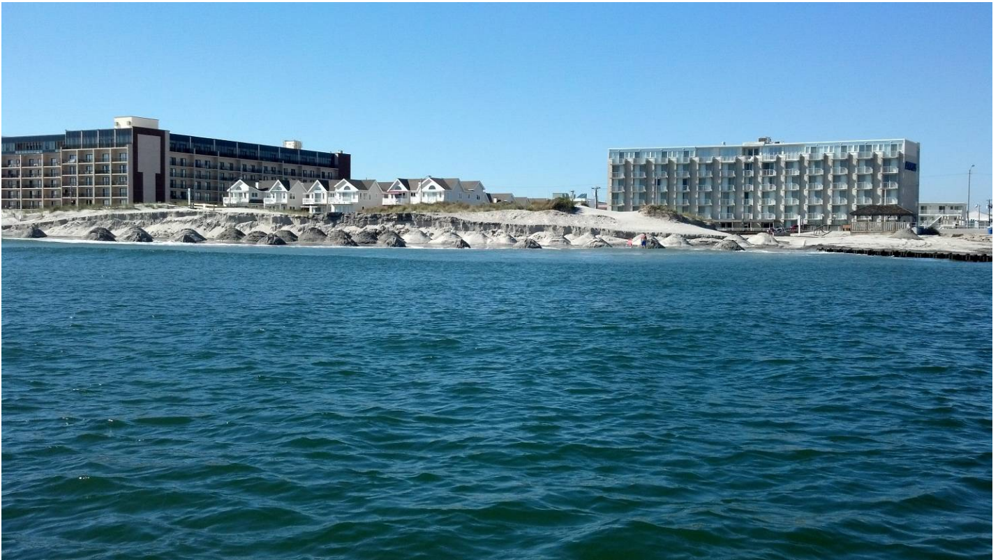
Figure 5. View from the ocean back to the combination of the sand piles placed on the beach and the material hauled back from Wildwood Crest's beaches to reinforce the dunes and widen the beach following Hurricane Irene as of May 2012.
