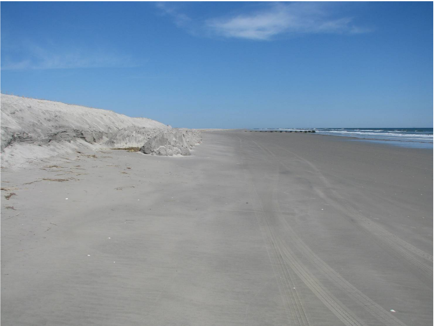
Figure 18. View of an early set of sand piles trucked north from the City of Wildwood provided from the excavation of the beach storm water discharge pipes that get buried in excess sand. The material is excavated and loaded onto North Wildwood trucks that drive north and drop the loads in a series making a row of piles at the toe of the dune scarp, then stagger the next row centered between the first row of piles. This cheap placement methodology works by making the wave swash rush up the piles, bounce between them and slow down far more rapidly than if the sand was graded into a flat slope up the scarp.
