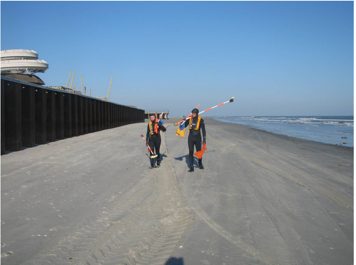
Figure 17. View to the north from where the dune crest at profile line location 64+00 existed pre-Sandy. High tide reaches the steel bulkhead every tide and the beach is as narrow as it was prior to the 2009 project. Although sand has accumulated in berm making the beach slightly wider, there is a need for restoration fill here in spite of the difficulty in maintaining any type of dune feature. The source of sand from the two communities down-beach is problematic at present, but perhaps communications and agreement can be achieved over time.
