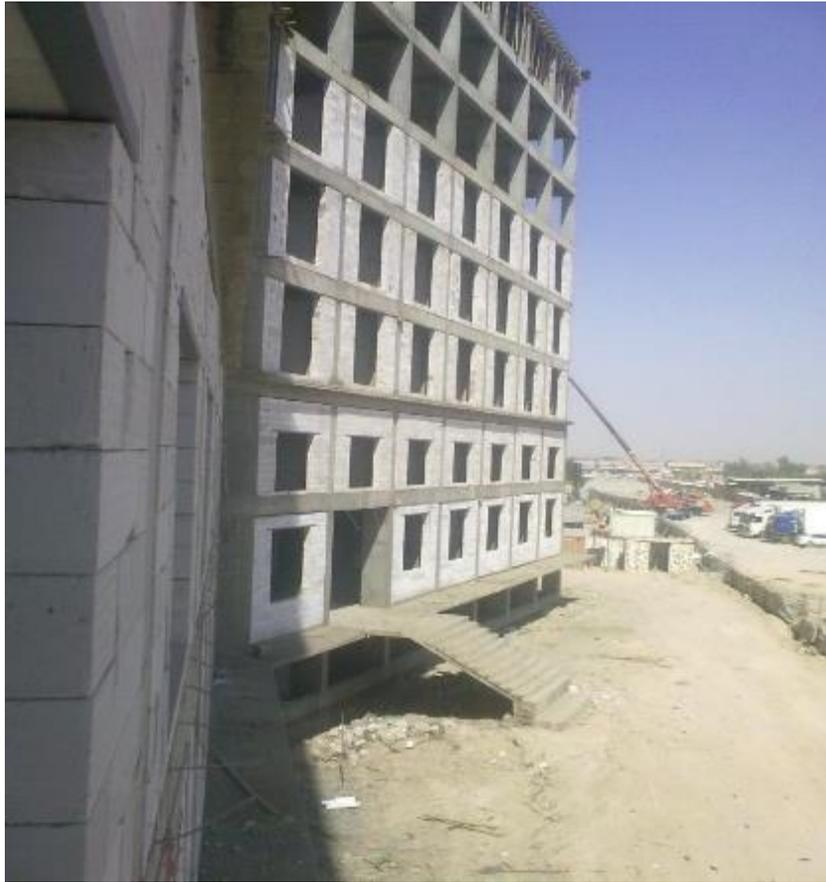
Figure 3. 1 AAC used as an exterior non-bearing wall in Najaf, Iraq
