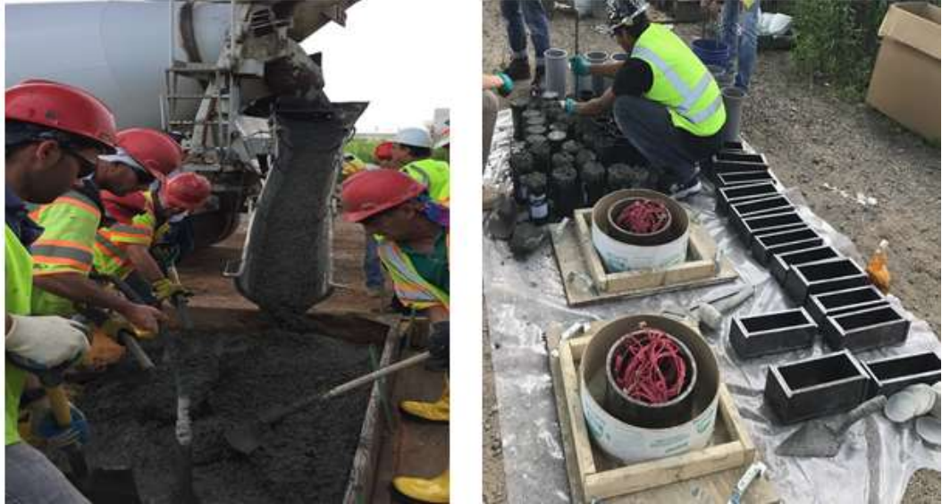
Figure 5.1 Casting of the Trial Slab and Field Sampling
