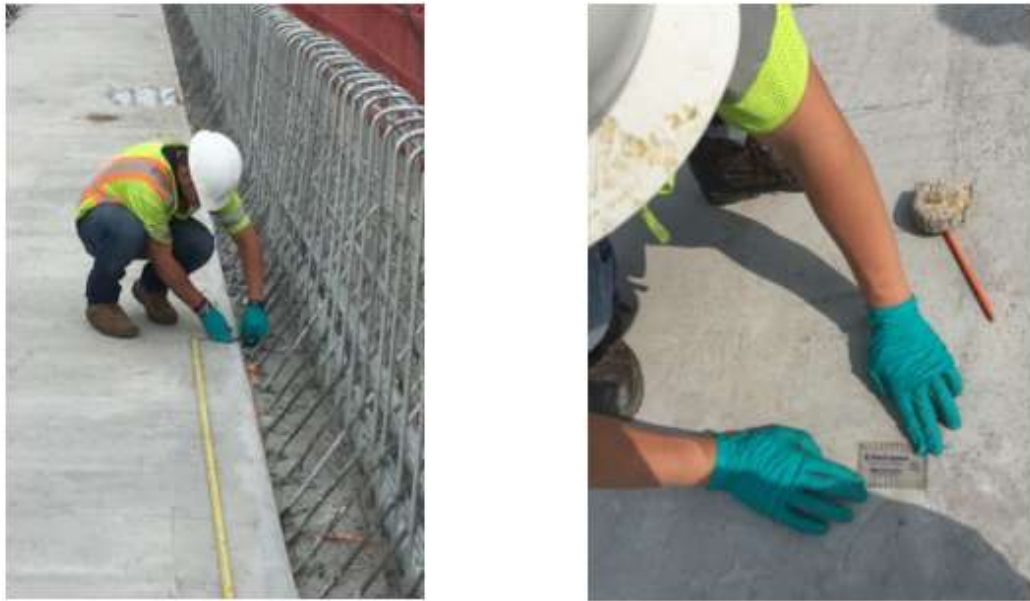
Figure 5.2 Crack Mapping
