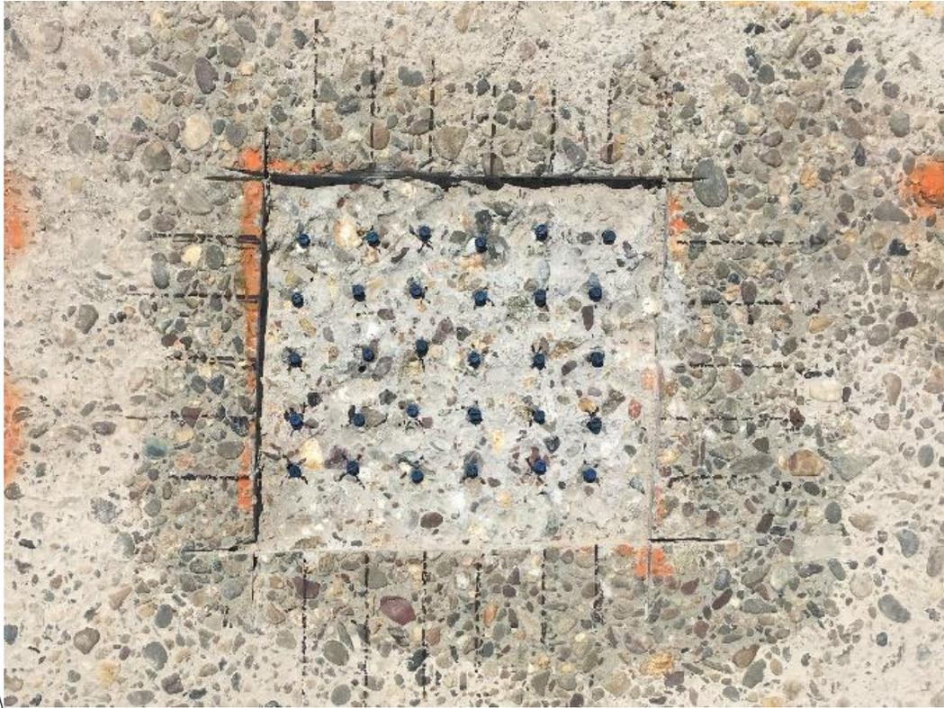
Figure 5.4 – Type 1 Mechanical Anchor Installation
