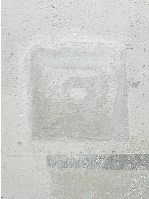
Figure 4.12 – Non-Horizontal Surface Repair: After Completion of Repair
