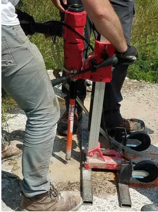
Figure 5.6 – Core Drill and Wet Core Bit Used to Make Circular Cuts
