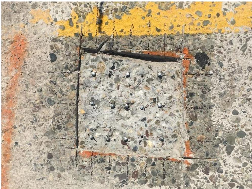
Figure 5.5 – Type 2 Mechanical Anchor Installation
