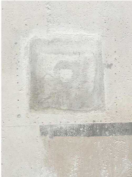
Figure 4.13 – Non-Horizontal Surface Repair: Two Years After Completion of Repair
