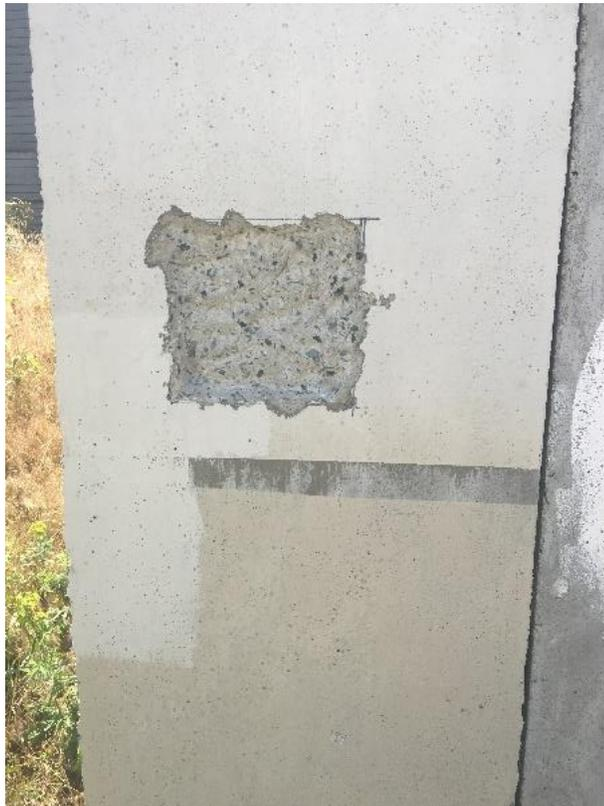
Figure 4.10 – Non-Horizontal Surface: Before Repair
