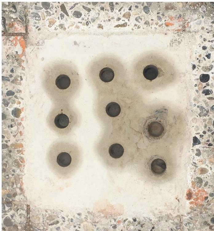
Figure 9.13 – RSHPR Patch Repair: 10 Months After Placement
