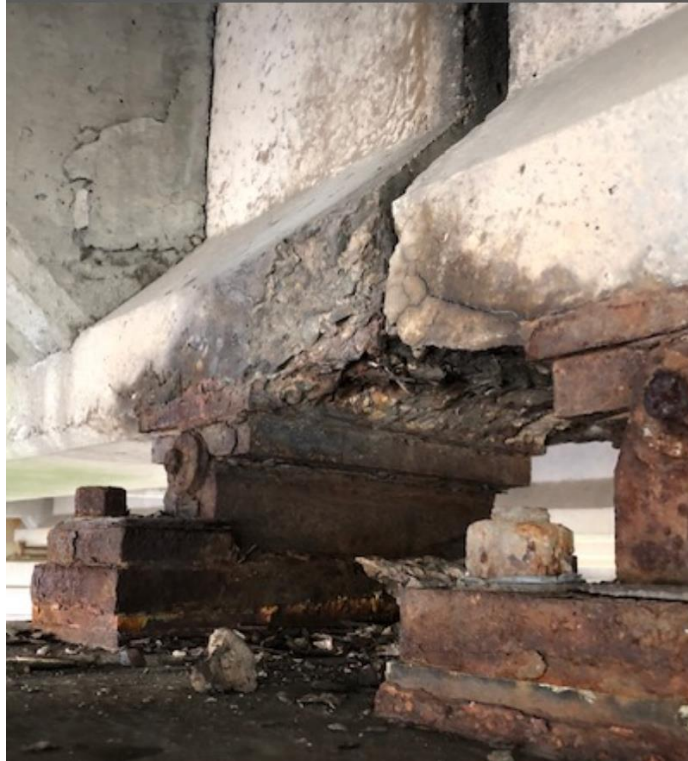
Figure 59. Deterioration at Support
